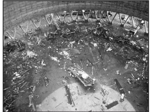
calculated stress resultants at several points in that part equaled or exceeded the strength of the shell in compression, bending and shear. The failure of these points in that part of the shell would have propagated to cause the collapse of the entire lift 28.
