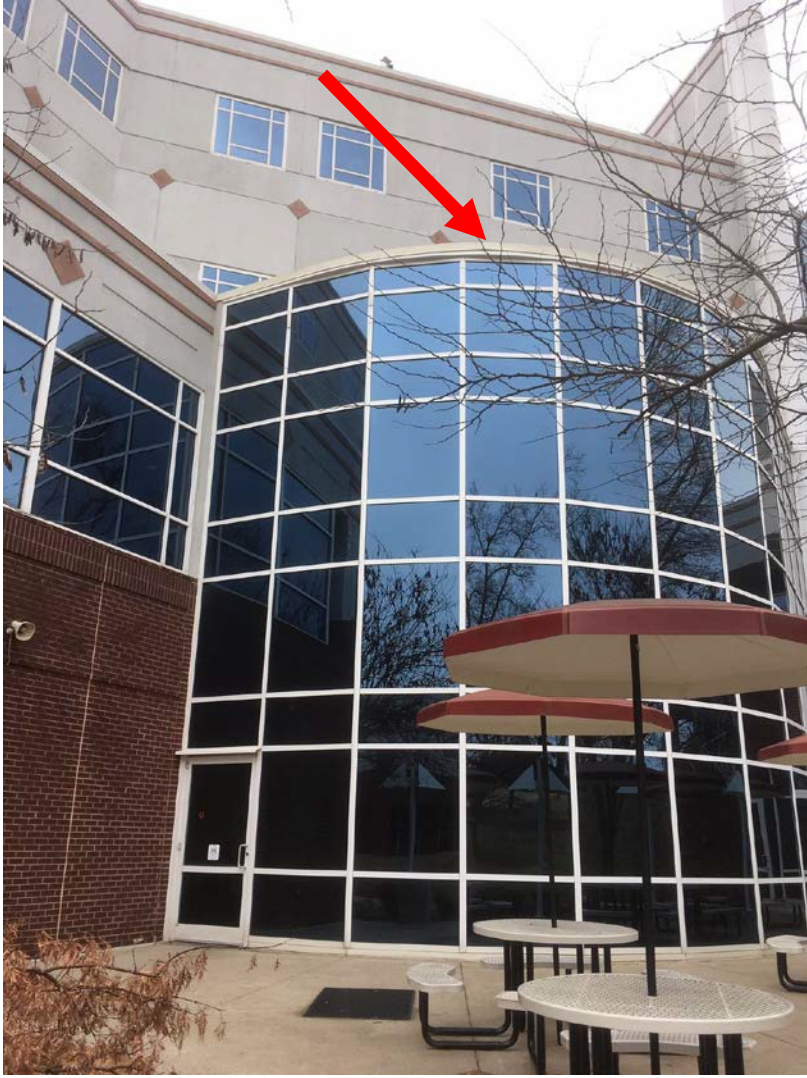
24 Fall from roof--Inspection #1451196 Ana Marquez dba H & M Cleaning & Painting
