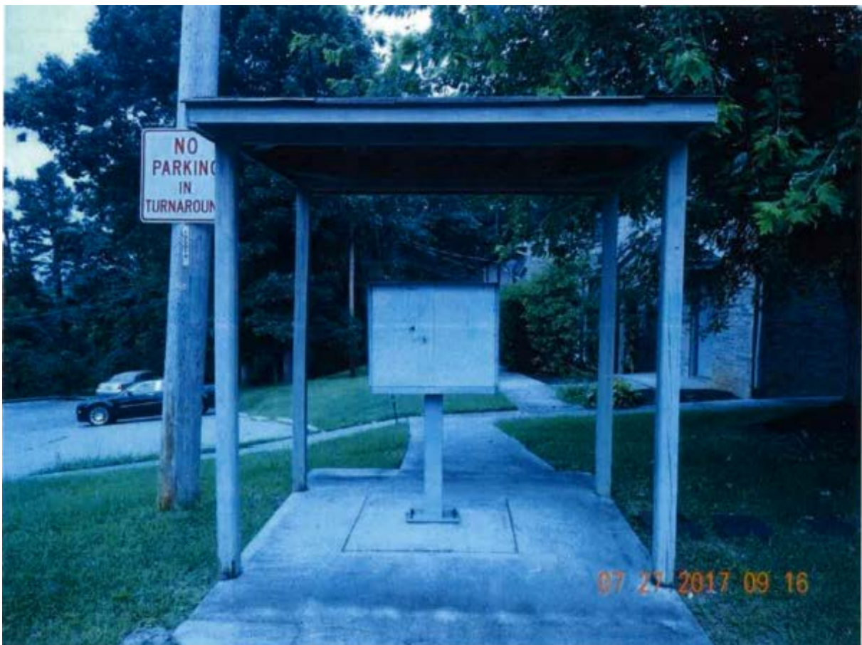
Photo 1 of 1 – A sidewalk leads from approximate location of parked FedEx truck to a dwelling near the end of the sidewalk. The wasp nest was located in the roof of the shed-like construction shown in the photo.
