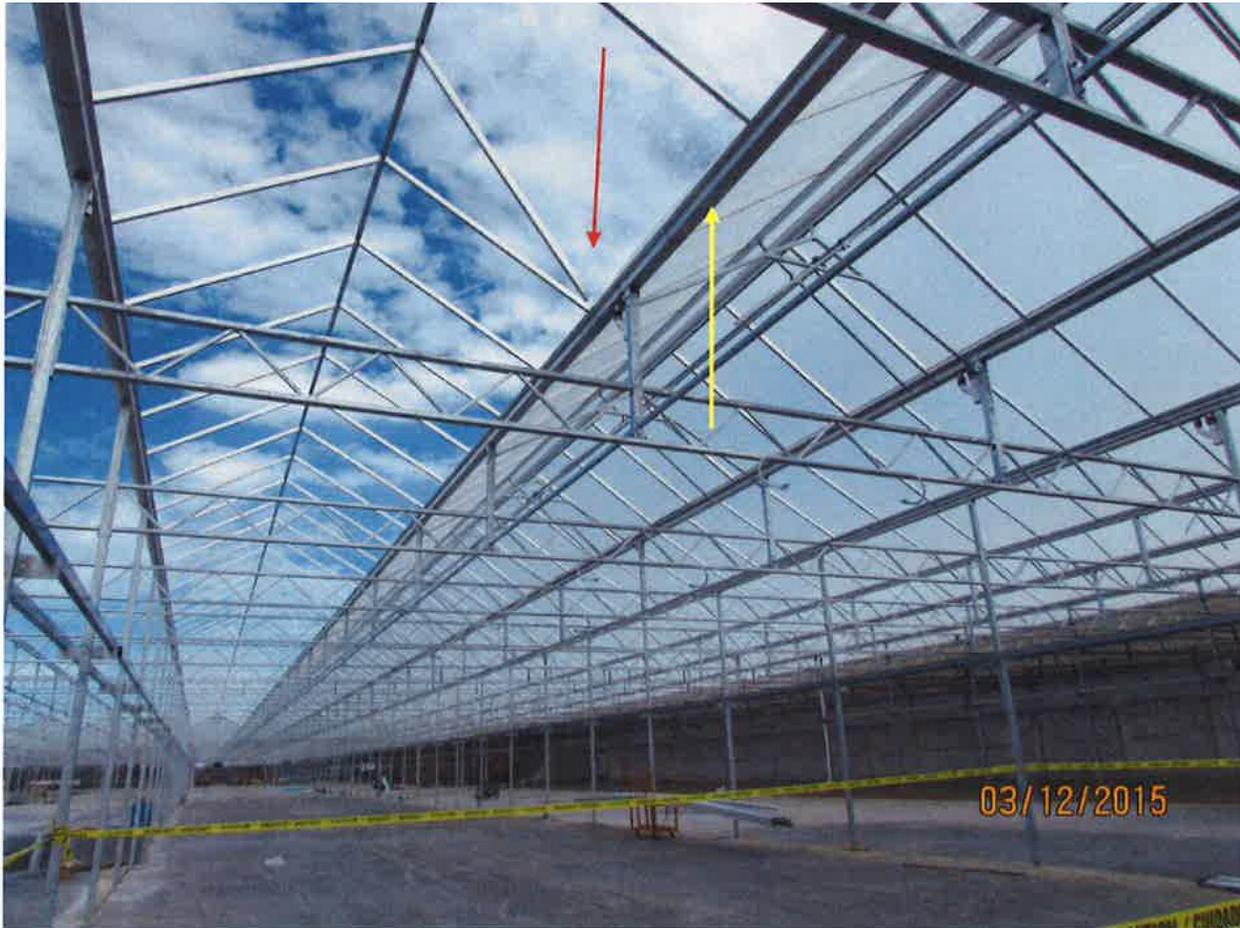
Photo 1 of 1 – This photo shows the gutter (yellow arrow) employees were standing on at the roof line, and a brace (red arrow) the victim broke during his 16 foot fall to the ground.
