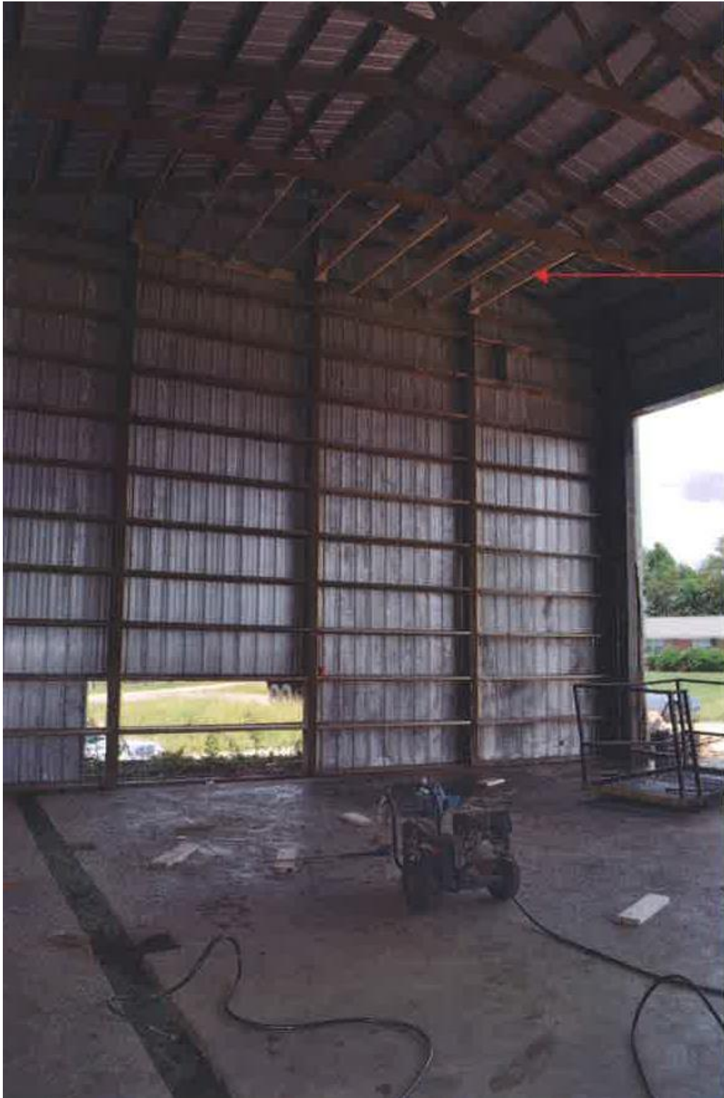
Photo 1 of 3: Ceiling to be erected by the contractor.
