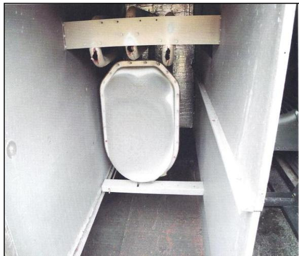
Inside heating unit where heat exchanger burned through pipes
