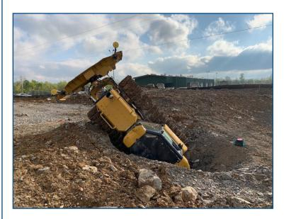
While working at a construction site in Middle Tennessee, a site contractor was performing grading work on a bioretention pond when he unknowingly backed his dozer off into an inlet to the pond that had already been dug but left with no markings or barricades. The dozer operator was wearing his seat belt and was able to walk away from the incident without injury.
