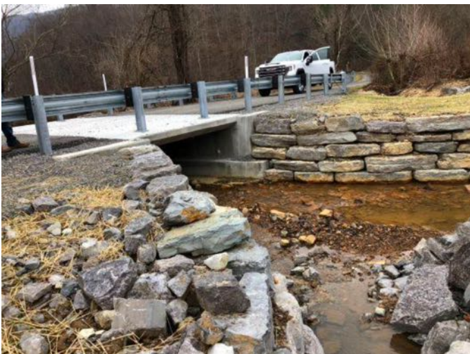
A severe barrier situation was addressed by replacing a culvert with a concrete bridge and box to allow more water to flow through the culvert in a more natural way / Robby Cogburn, Partners for Fish and Wildlife, USFWS
