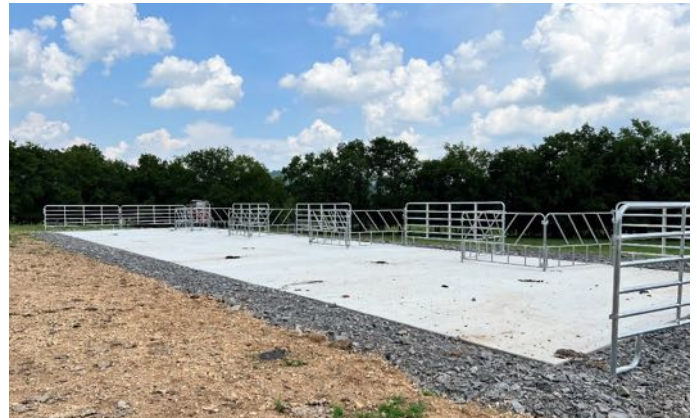
Two new heavy-use area concrete feeding pads, cross fencing, alternative water sources, and an access road allow the landowner to rotate his cattle more efficiently throughout the year. With feeding pads on either side of the creek, the landowner can move his herd across a stabilized creek crossing. /Lauren Neale, TN Cattleman's Association
