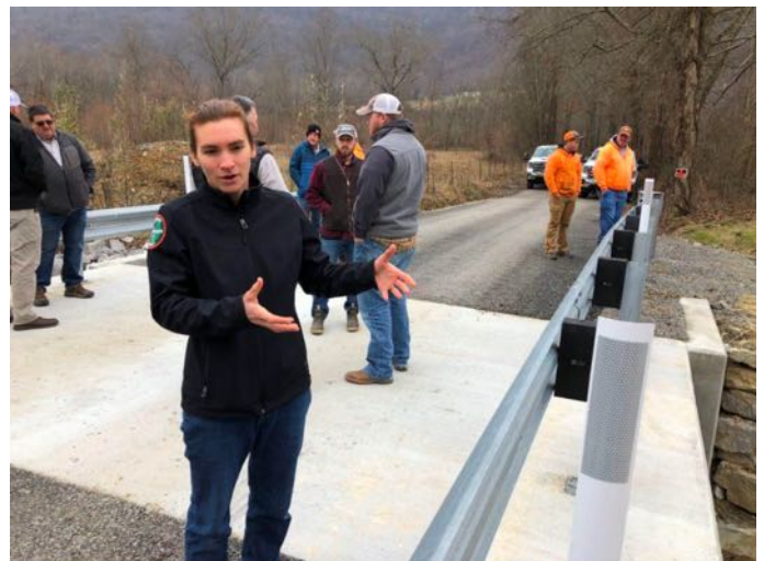
TWRA Fish Biologist Sally Petre explains that the wider bridge compared to the old narrow culvert it replaced allows more water flow, which is good for the fish and reduces flooding. — formerly a common occurrence / WLAF News
