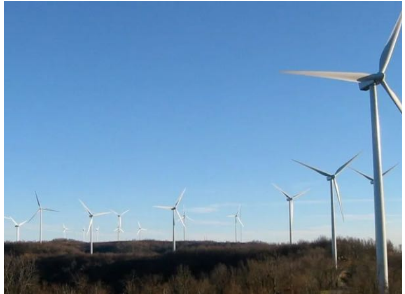
Buffalo Mountain wind farm / Tennessee Valley Infrastructure Group
