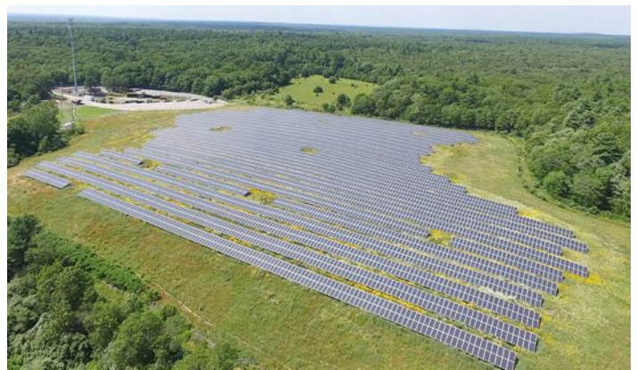
Solar array on top of a former landfill / Wikimedia
