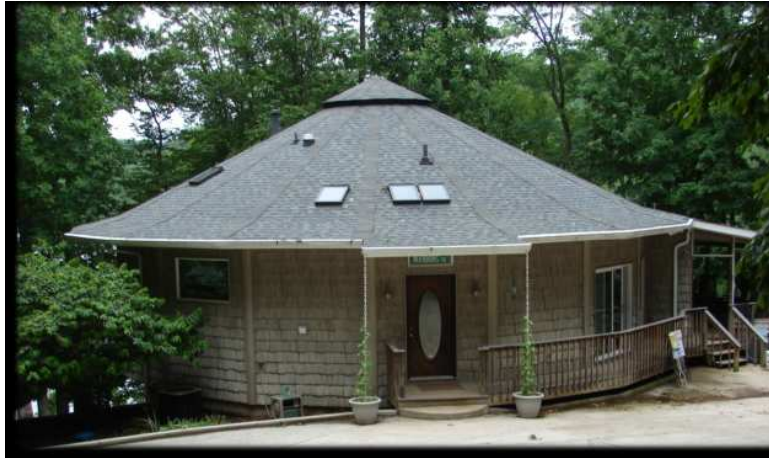
Newer Construction with Vinyl Siding and Asphalt Shingle Roof
