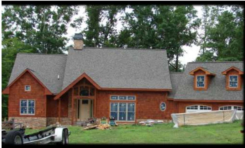
New Construction with Wood Siding and Asphalt Shingle Roof
