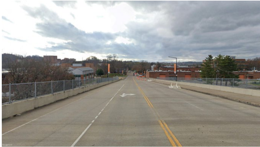
Joe Johnson Drive - Existing
