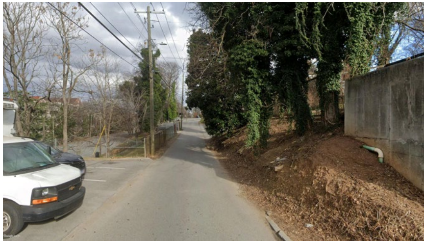
Caledonia Avenue - Before
