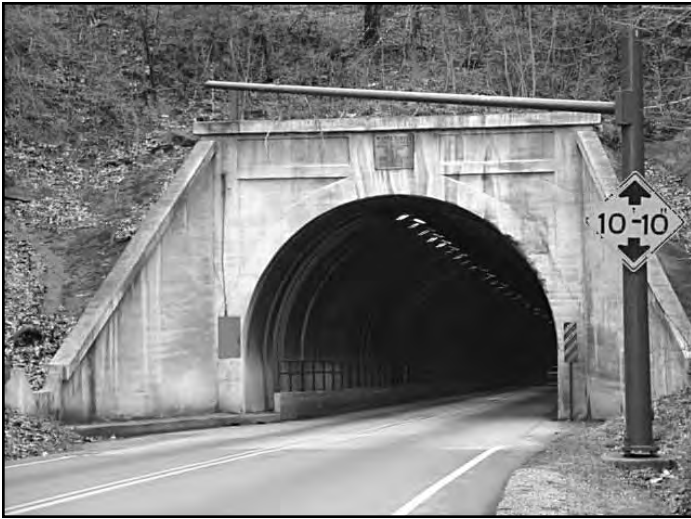
Figure I-05: View of the 1929 Wilcox Tunnel through Missionary Ridge in Chattanooga.
