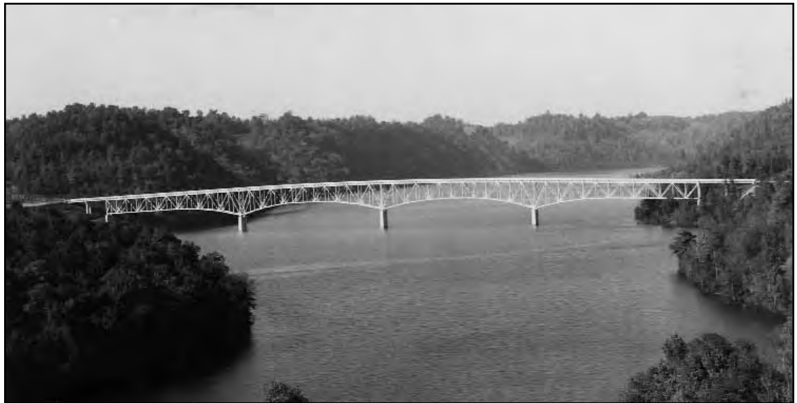
Figure 1-06: Postcard view of the Hurricane Creek Bridge across Center Hill Lake in Dekalb County. The Army Corps of Engineers erected this continuous truss in 1948-1949. It is not included in the survey since it was built after 1945 (Author's Collection).
