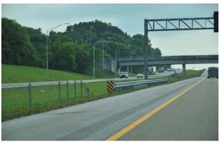
A pre-installation review should have found that this placement of two end terminal resulted in a gap in the median shielding and recommended an overlapping design treatment.
