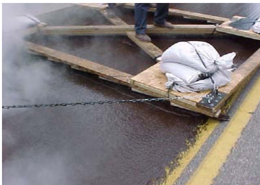
Ribbon of material in front of broom
