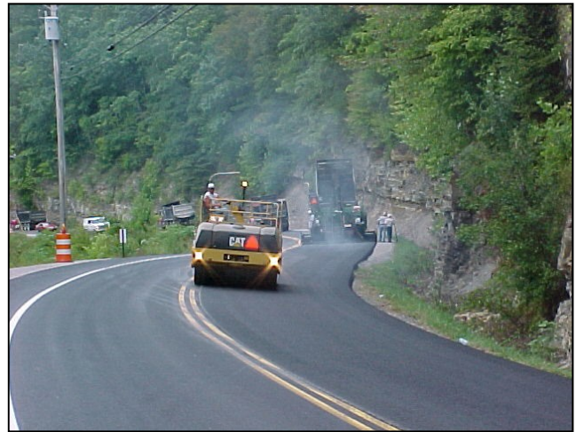
DeKalb County - SR 26 – Binder (BM-2) Placement
