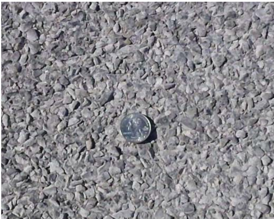
Chip Seal prior to Microsurfacing Lift being placed
