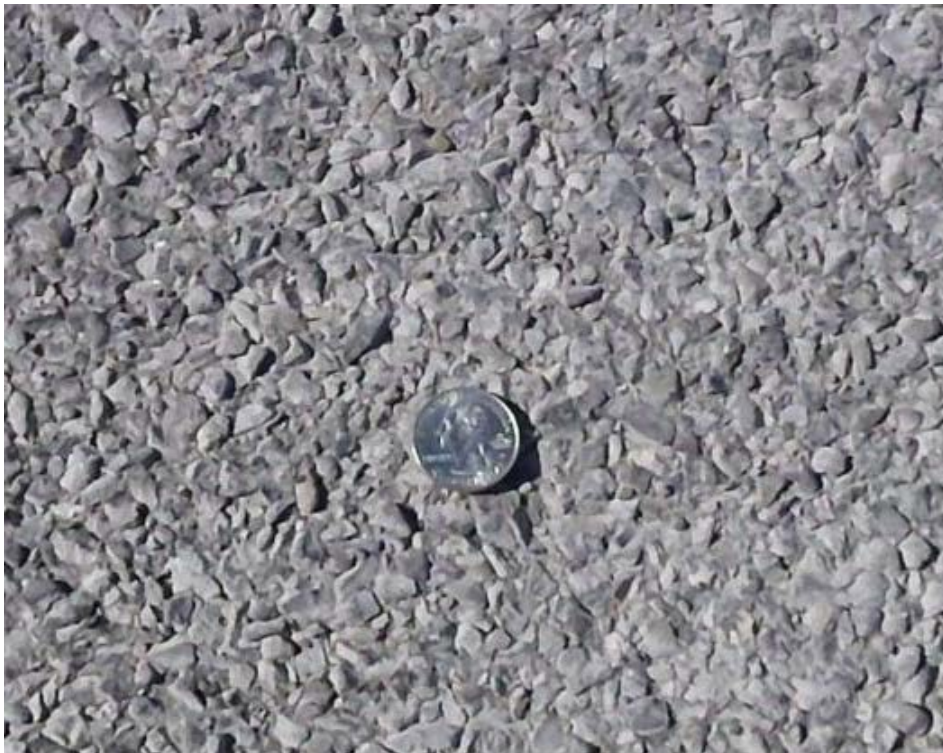
Chip Seal prior to Thin Lift of Hot Mix Asphalt being
