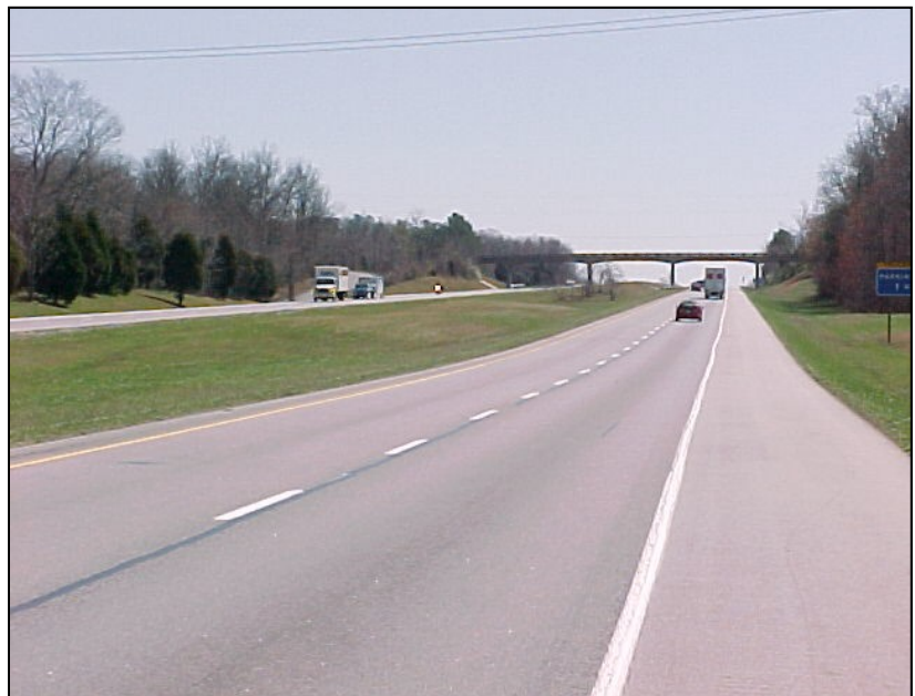
Centerline joint sealed
