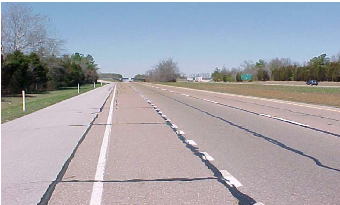
Quantity of crack seal is excellent; however, longitudinal crack seal is too heavy.
