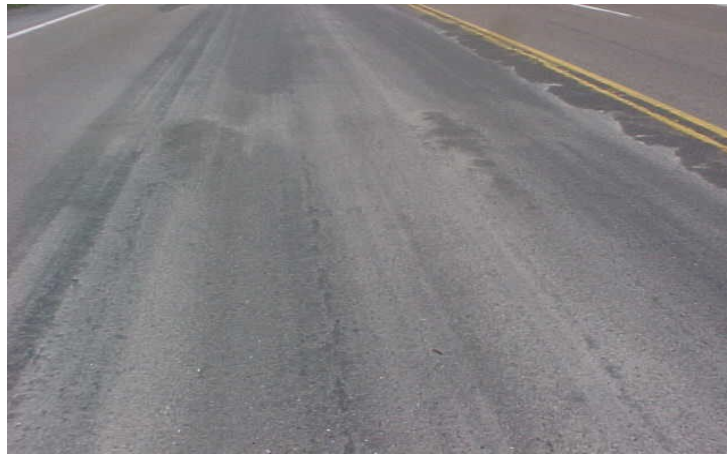
Scrub Seal approximately one year after placement salt is present from winter treatment
