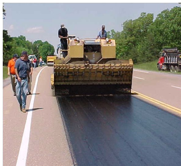
Aggregate applied to asphalt
