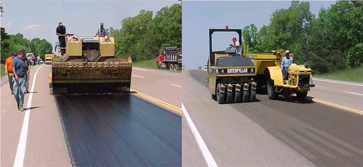
Aggregate applied to asphalt sealer Rolling of aggregate cover material – 2 passes
