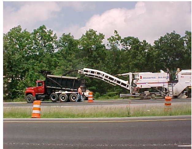
Milling machine in operation
