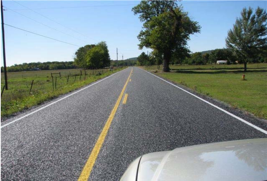
Completed Chip Seal w/ Fog Seal
