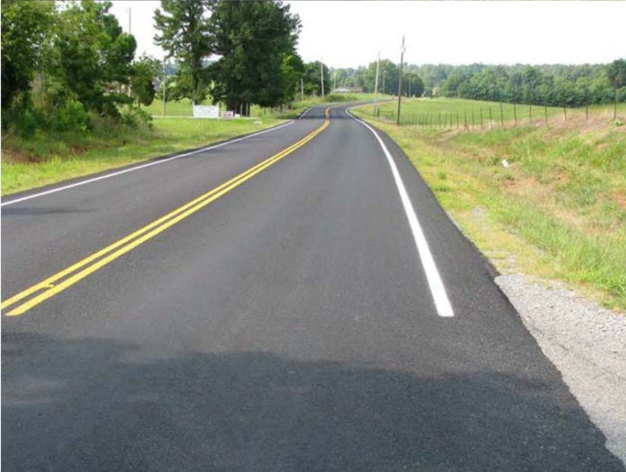
Completed Chip Seal with 24 lbs/SY Microsurfacing
