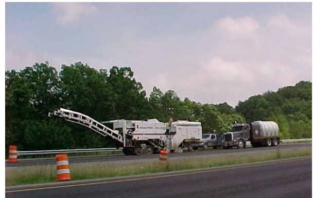
Milling Machine and Water Truck
