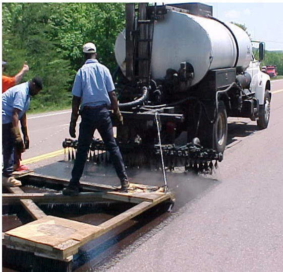
Application of asphalt sealer sealer
