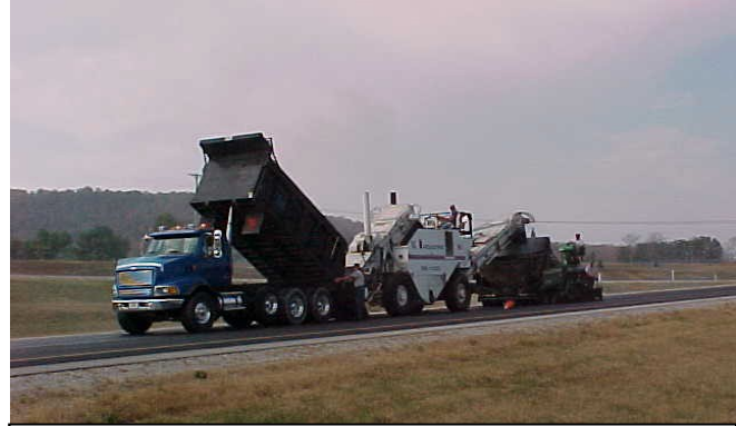
Use of shuttle buggy on thin overlay
