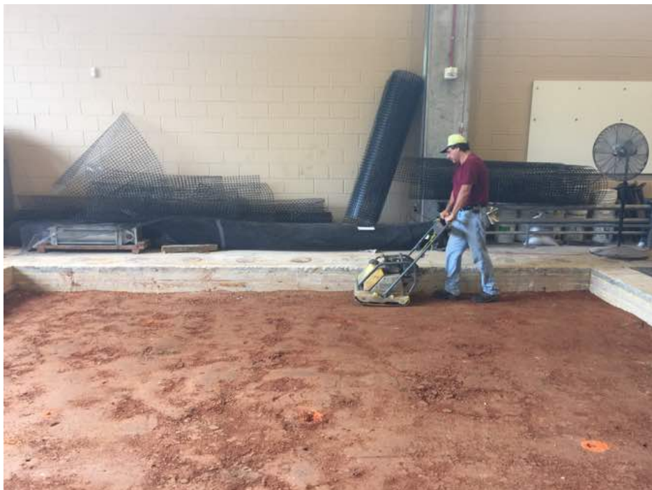
Figure 5.5: Compacting the Edge Area with a Hand-Held Vibrator
