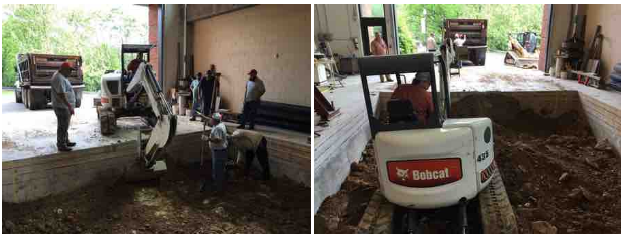
Figure 4.5: Placing Subgrade Soil
