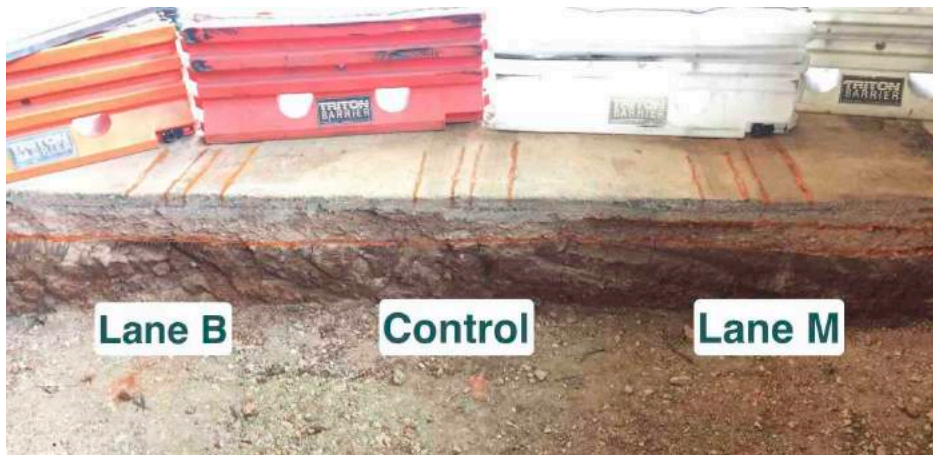
Figure 6.95: Resulted Cross Section from Trenching
