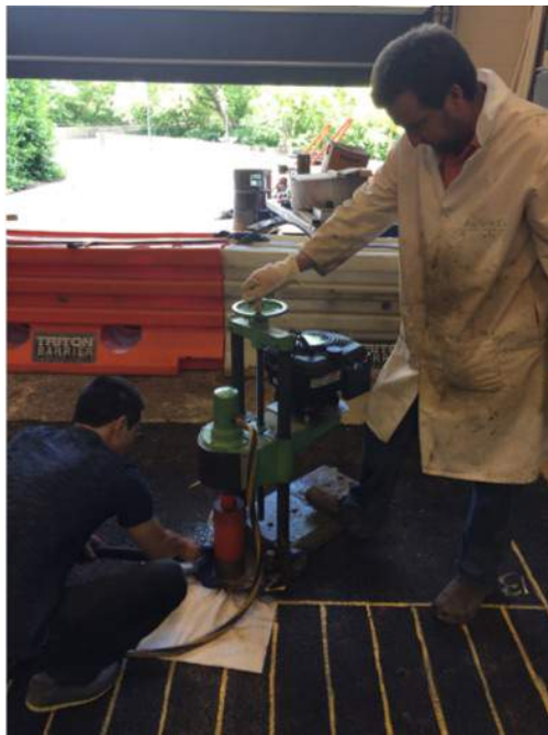
Figure 5.7: Coring Test Conducted to Verify Asphalt Layer Thickness
