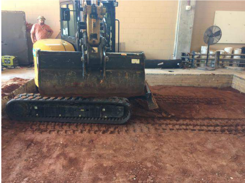
Figure 5.2: Pre-Compacting Refilled Subgrade Soil with a Caterpillar Excavator
