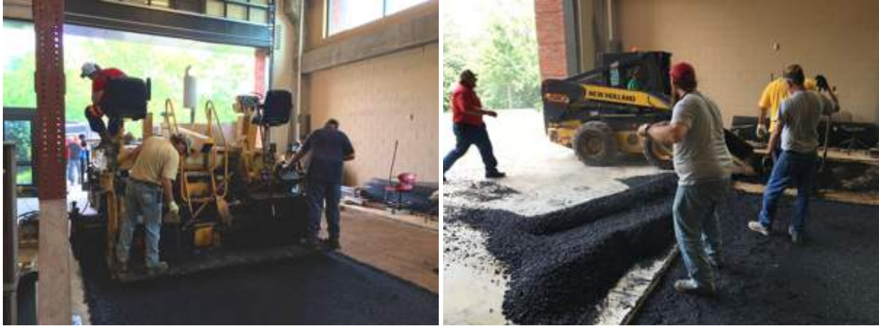
Figure 4.8: Placing Asphalt Mixture
