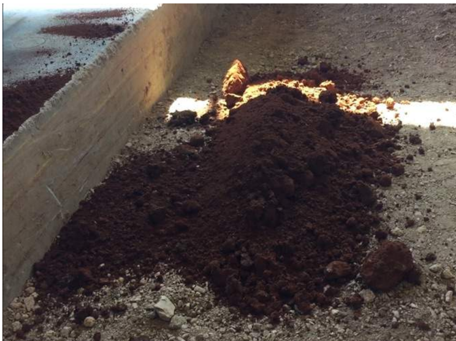
Figure 5.1: Refilling Subgrade Soil
