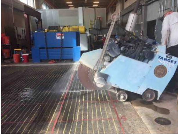
(a) Cutting Asphalt Layer
