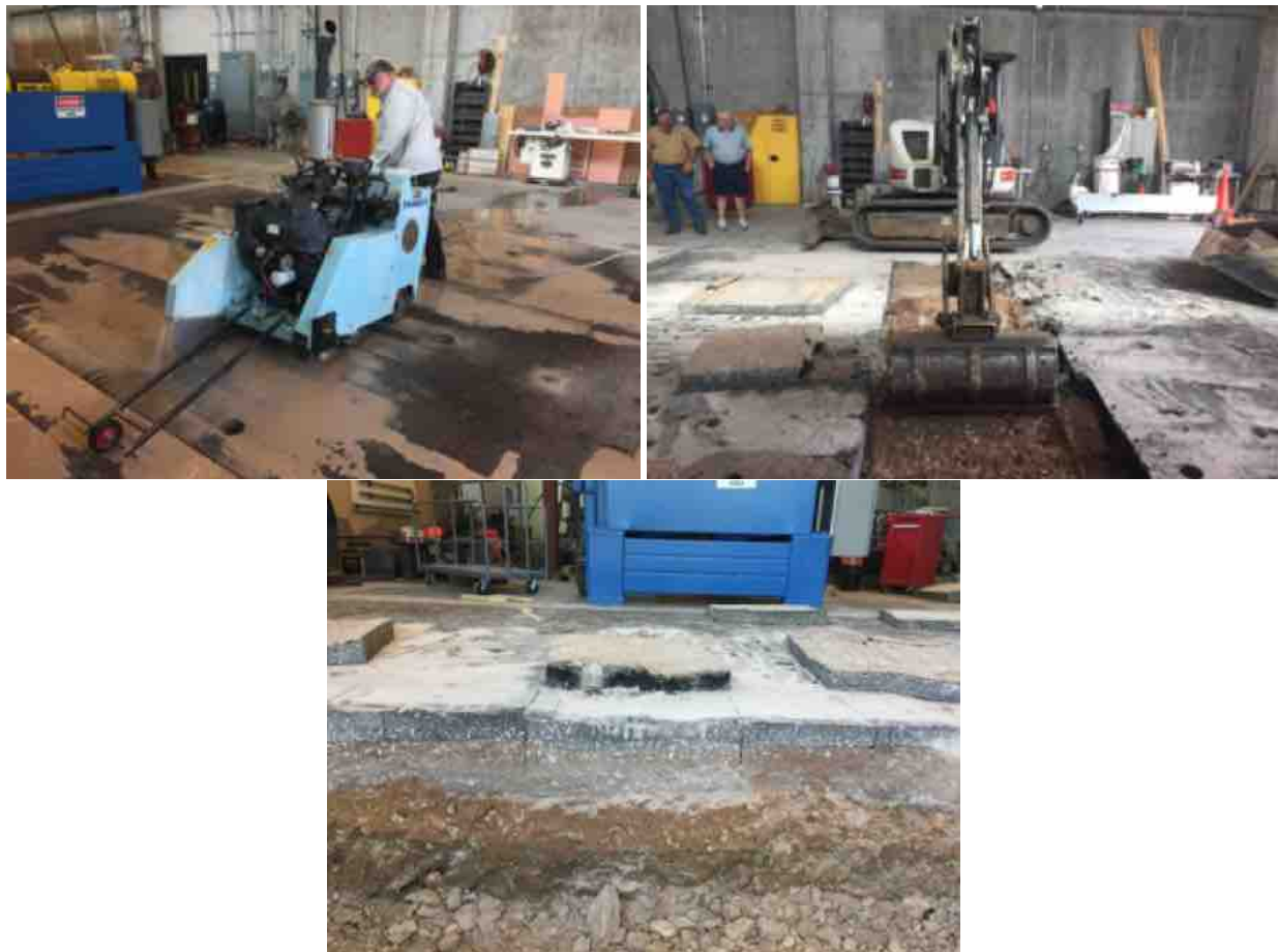
Figure 4.48: Overview of Cutted Test Pit (Round 1)
