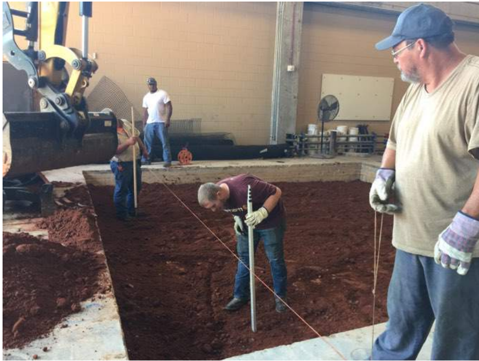
Figure 5.4: Controlling the Thickness of Subgrade
