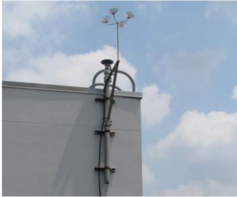
View mount attached to bldg
