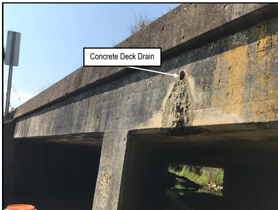
Photo 6: View of concrete deck drain on the SR-19 bridge over Briar Creek
