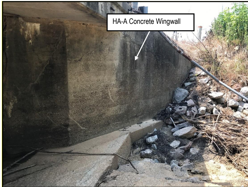
Photo 1: View of HA-A on the SR-19 bridge over Meridian Creek
