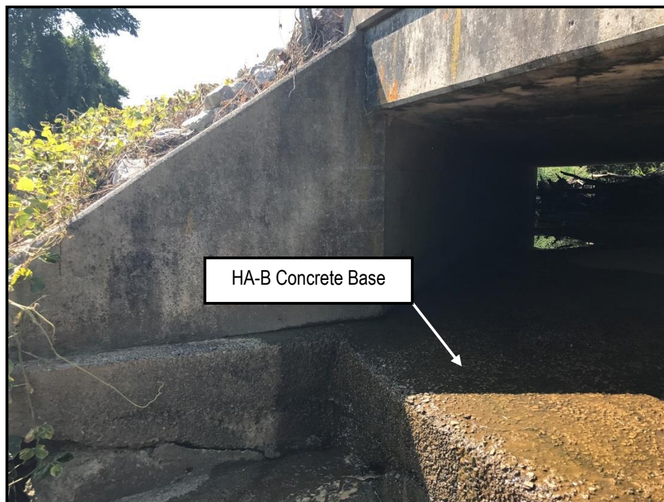
Photo 2: View of HA-B on the SR-19 bridge over Briar Creek
