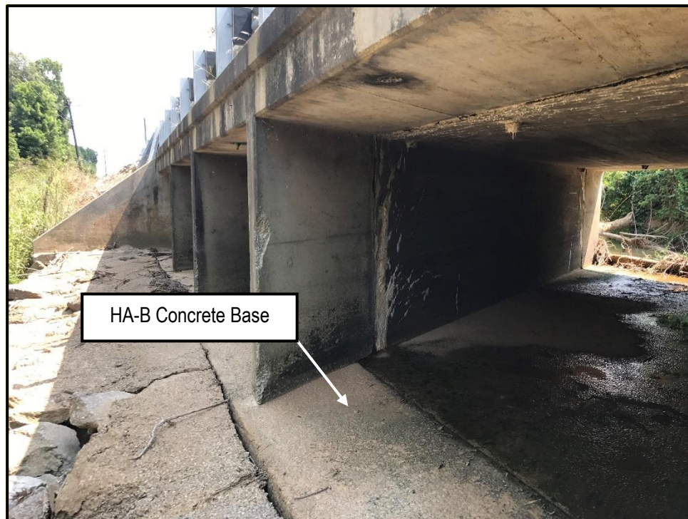
Photo 2: View of HA-B on the SR-19 bridge over Meridian Creek
