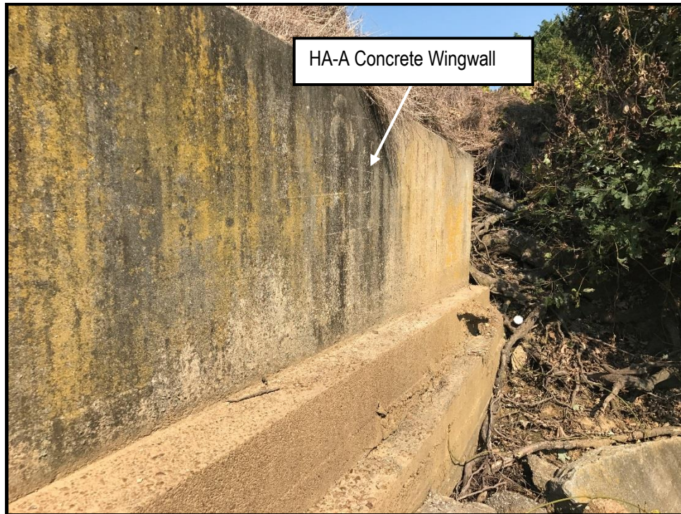
Photo 1: View of HA-A on the SR-19 bridge over Briar Creek
