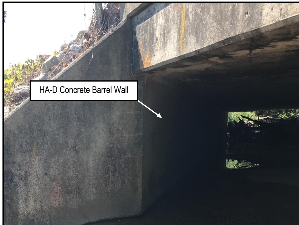
Photo 4: View of HA-D on the SR-19 bridge over Briar Creek
