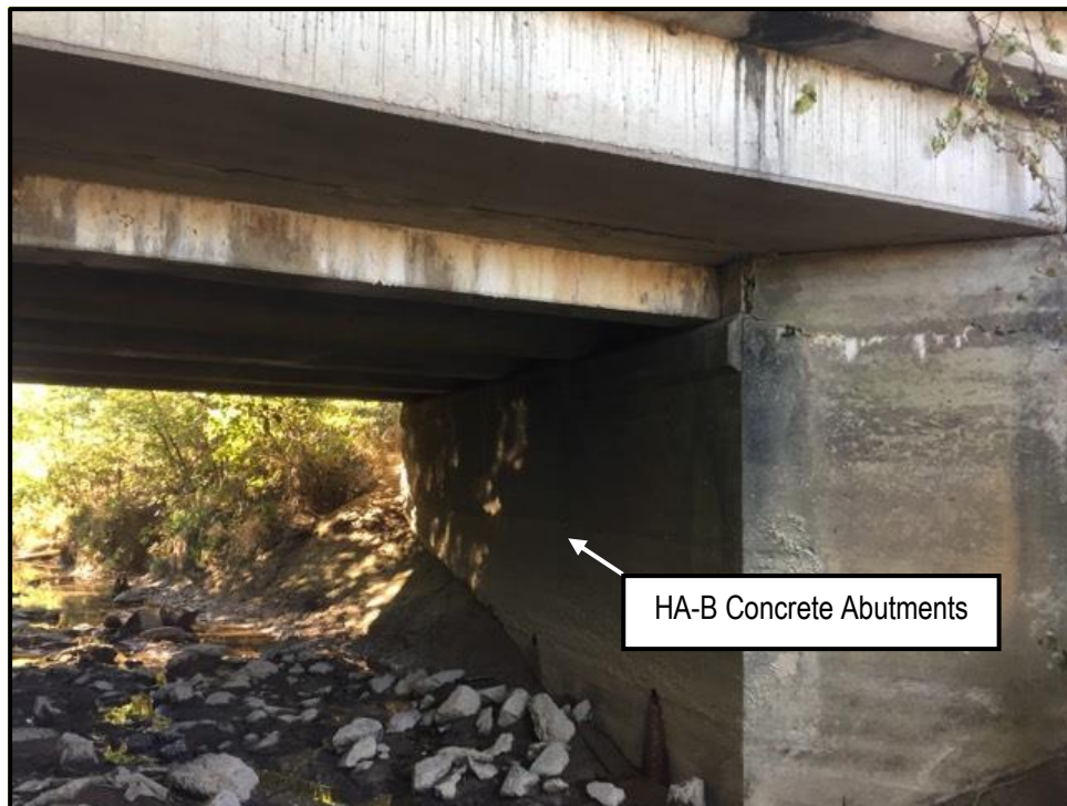
Photo 2: View of HA-B on the SR-19 bridge over Branch
