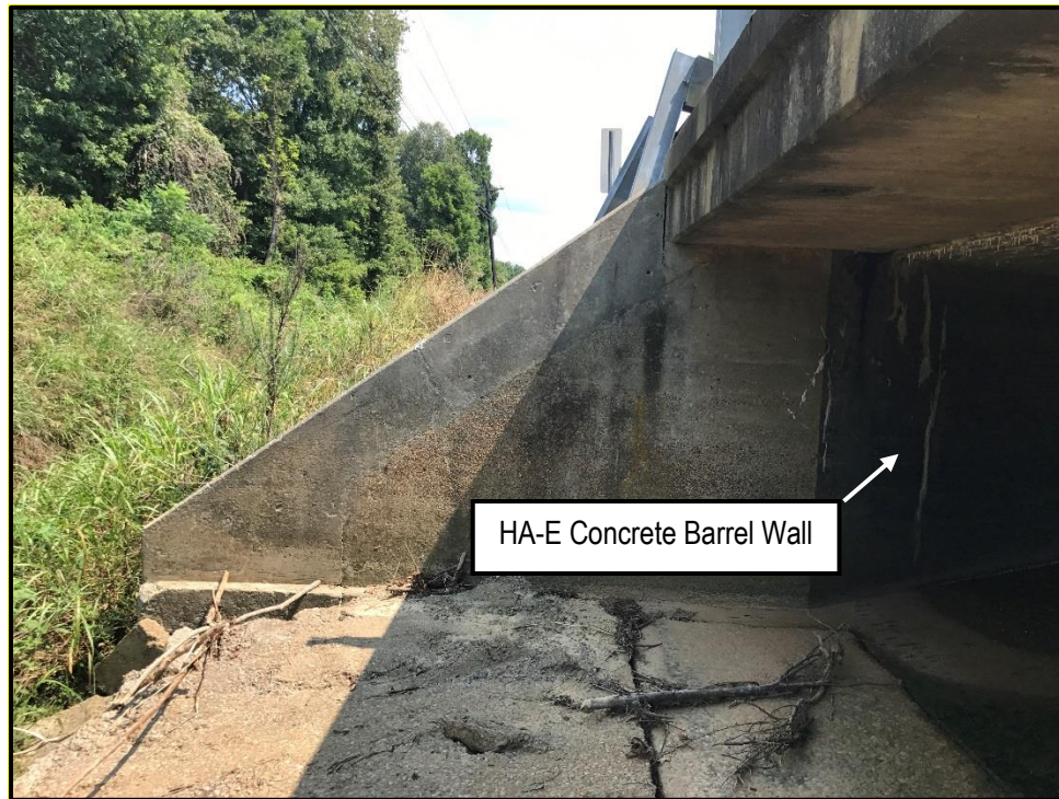
Photo 5: View of HA-E on the SR-19 bridge over Meridian Creek
