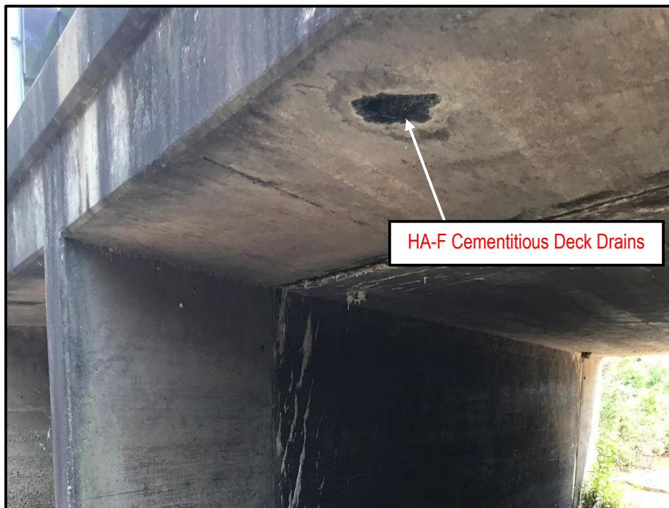
Photo 6: View of HA-F on the SR-19 bridge over Meridian Creek
