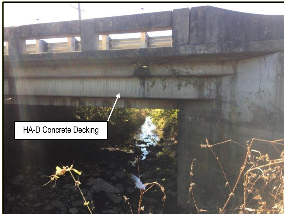
Photo 4: View of HA-D on the SR-19 bridge over Branch
