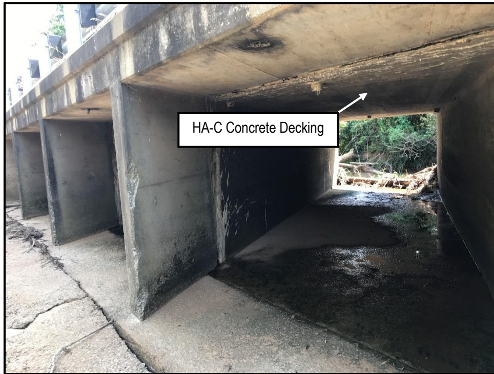
Photo 3: View of HA-C on the SR-19 bridge over Meridian Creek
