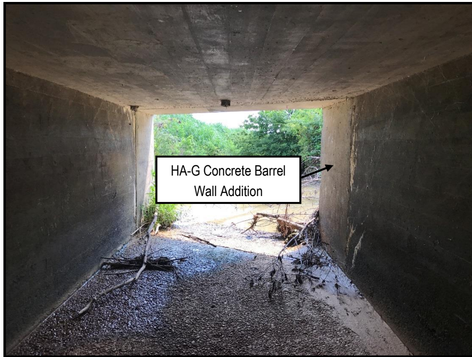
Photo 7: View of HA-G on the SR-19 bridge over Meridian Creek
