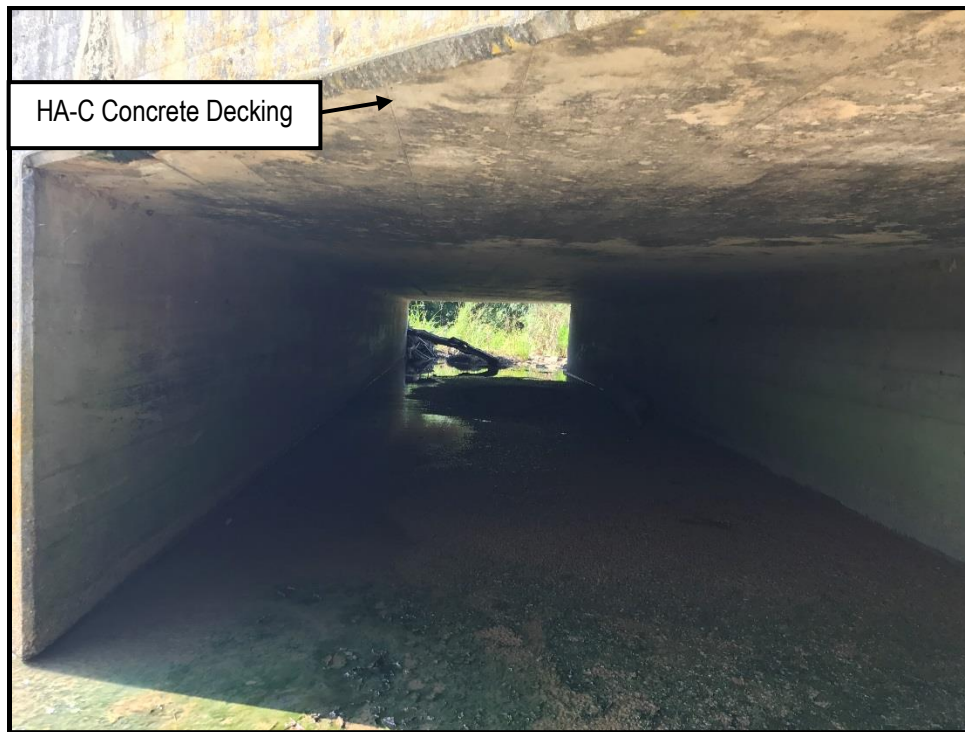
Photo 3: View of HA-C on the SR-19 bridge over Briar Creek
