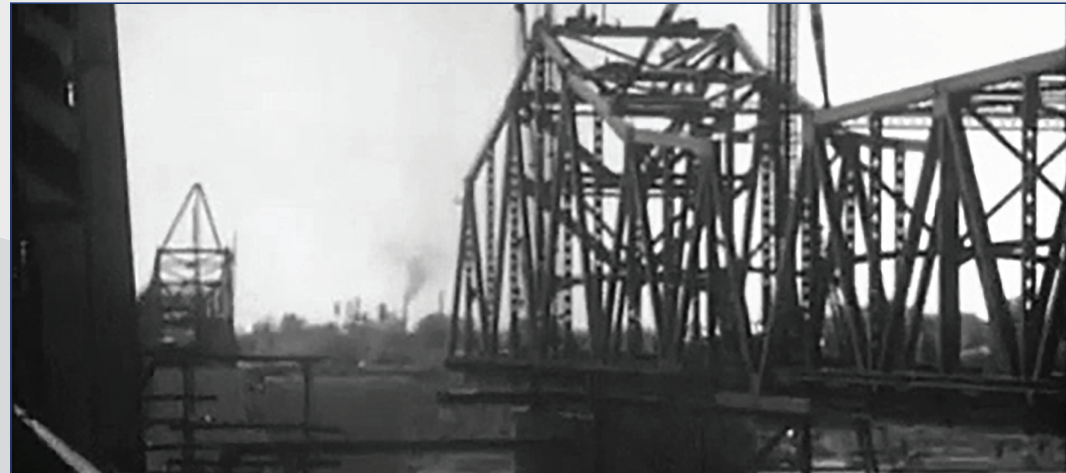
Bridge under construction in 1949
