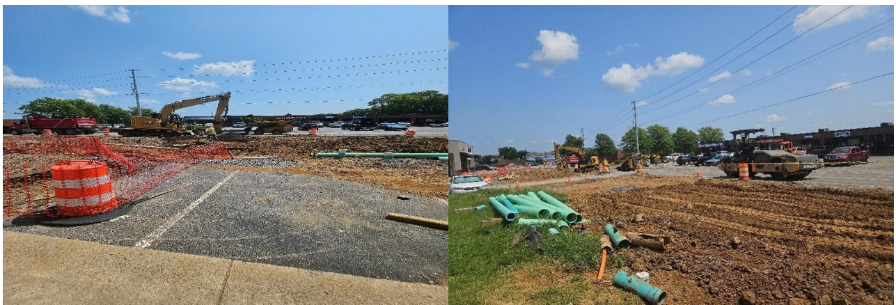
Traffic signal work.
