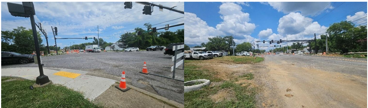
Traffic signal pole foundation installation.
