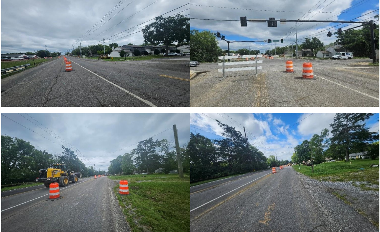
Traffic switch on Walton Ferry Road.
