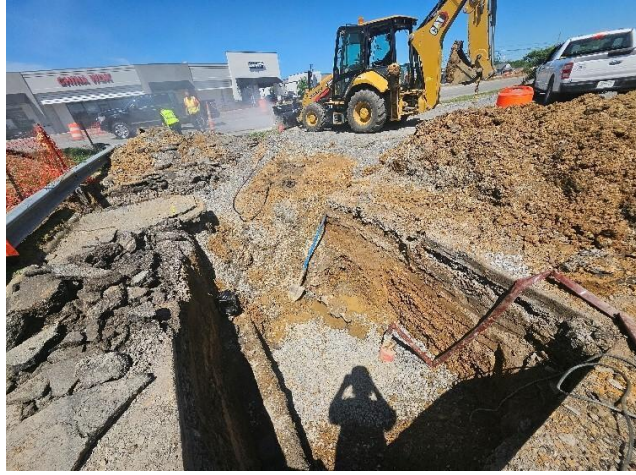
Water main connections.
