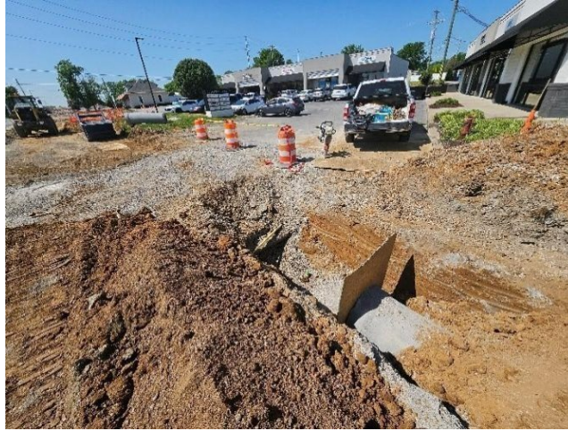
Storm drain installation.
