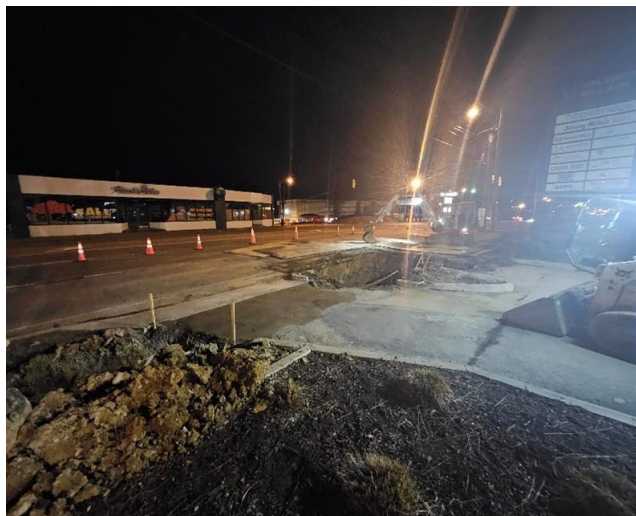
AT&T vault installation.
