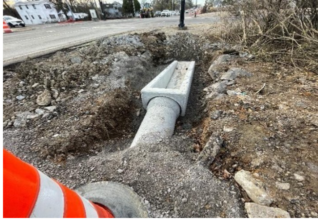
Storm drain installation.
