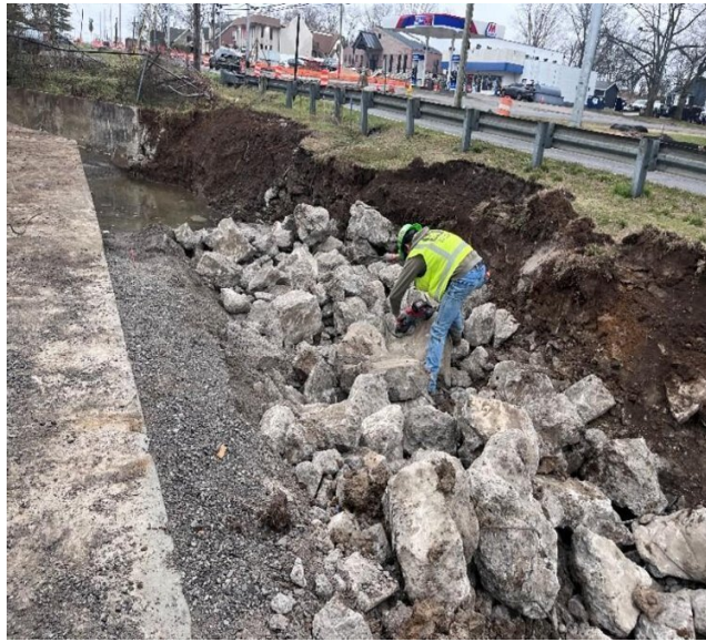
Box culvert demolition.
