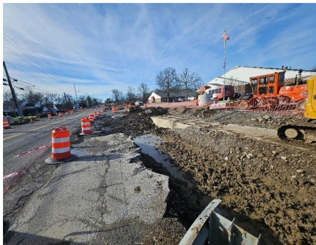
Box culvert backfilling.
