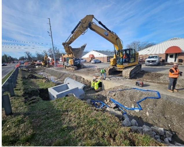
Storm drainpipe installation
