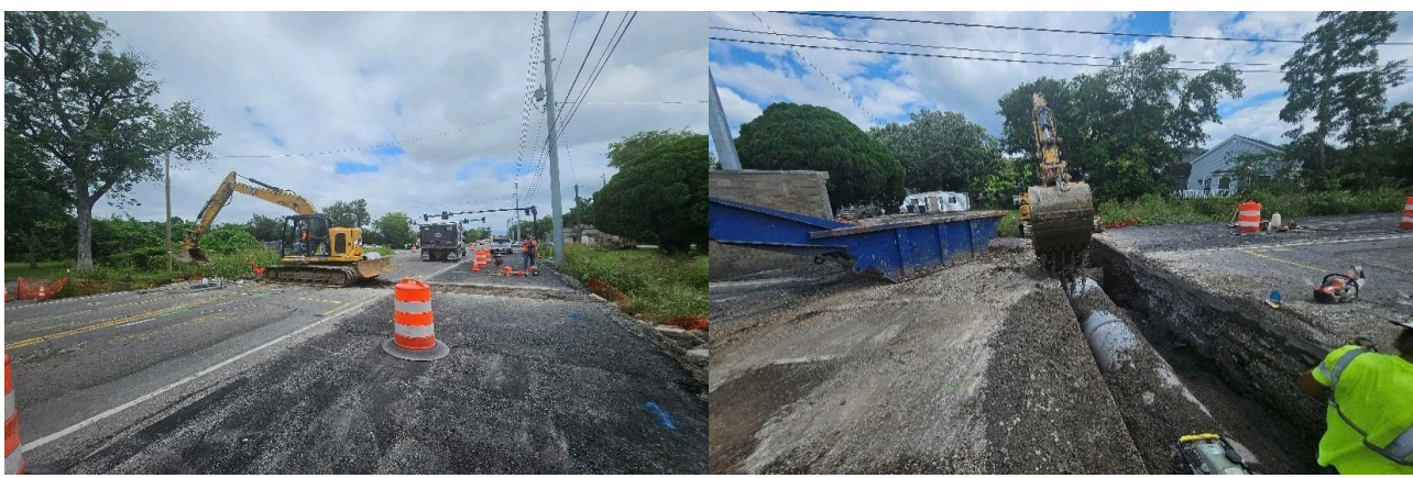
Storm drain installation.
