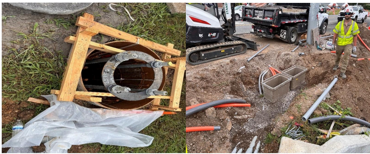
Traffic signal pole foundation installation.
