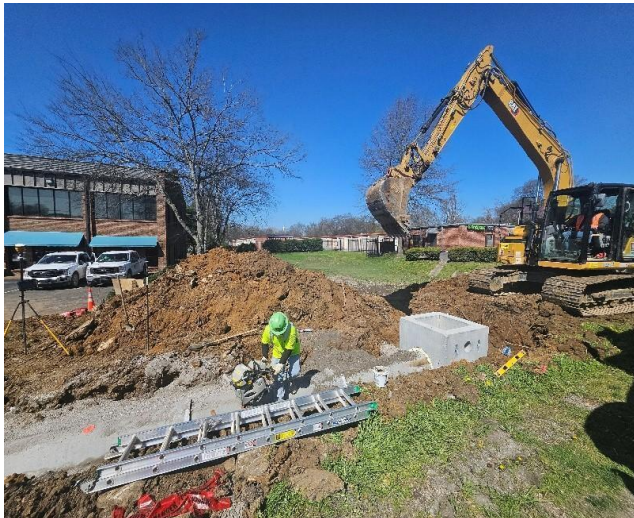
Storm drain installation.
