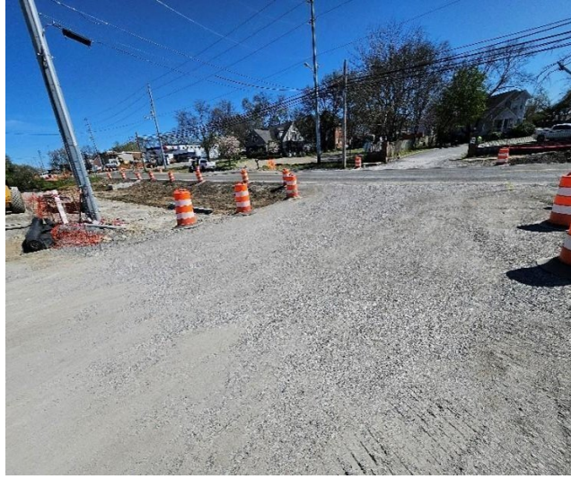
Box culvert backfill.
