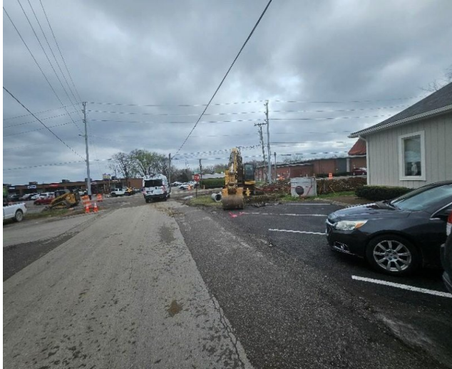
Storm drain installation.
