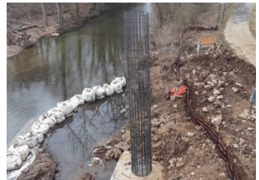
Steel for one of the new bridge piers.
