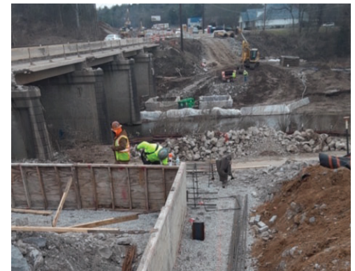
Bridge widening work at Whites Creek.
