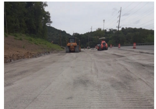
Widening on Clarksville Pike near Kings Lane.
