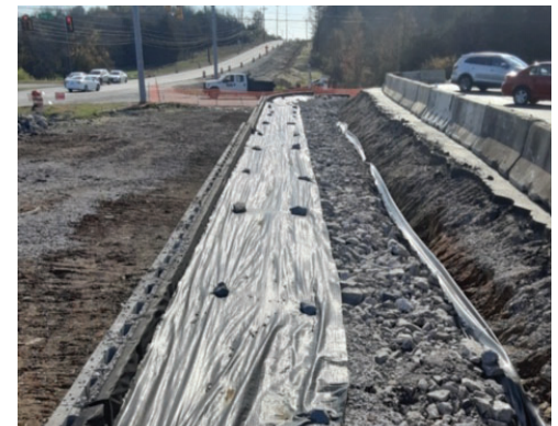
Retaining wall work on Clarksville Pike.
