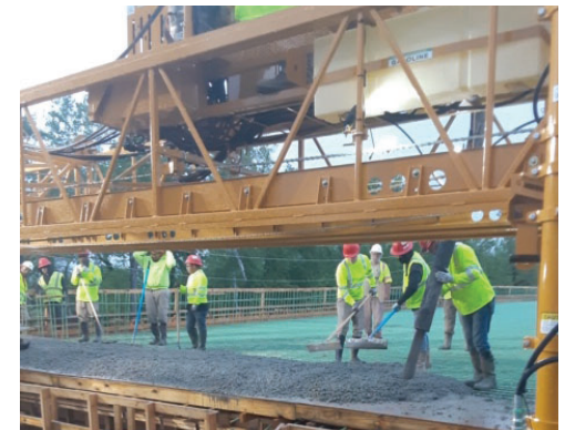
Bridge widening work at Whites Creek.
