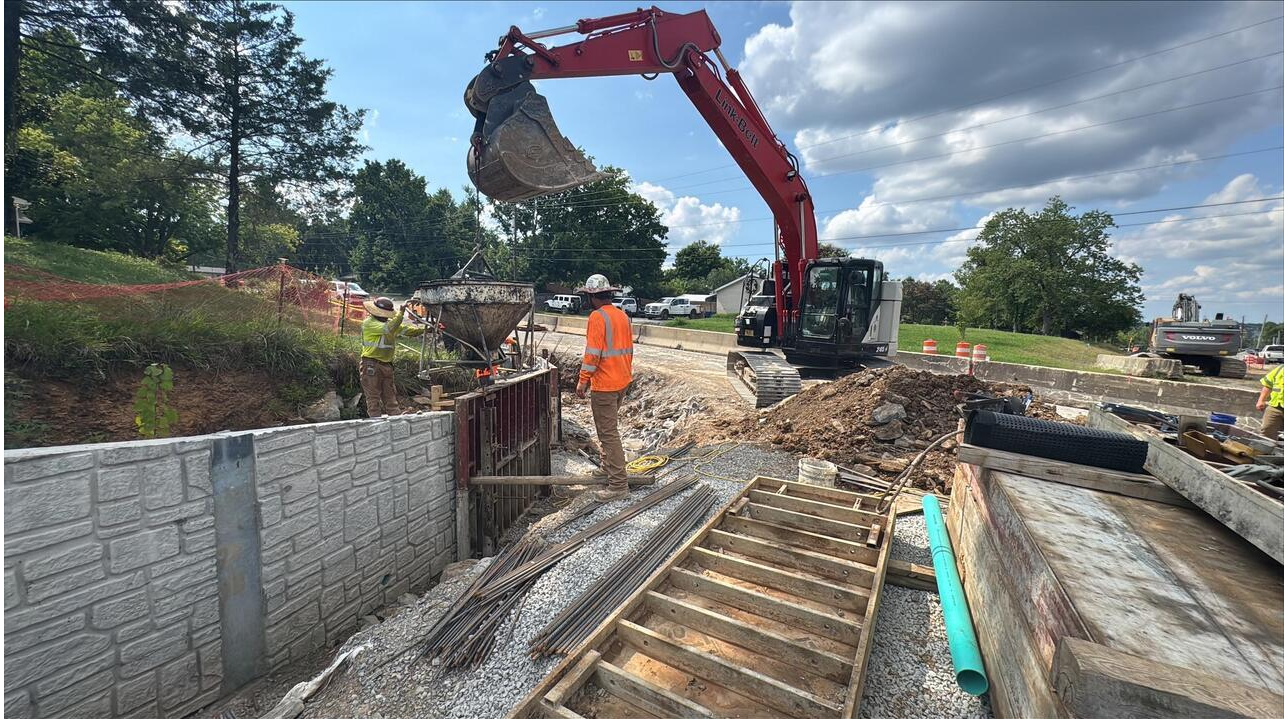
Retaining wall 2 completion.
