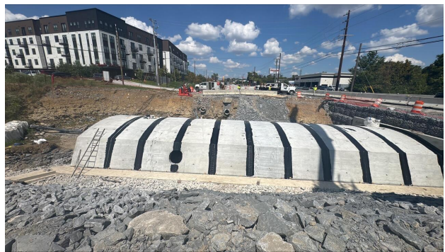
Mainline arch culvert placement.
