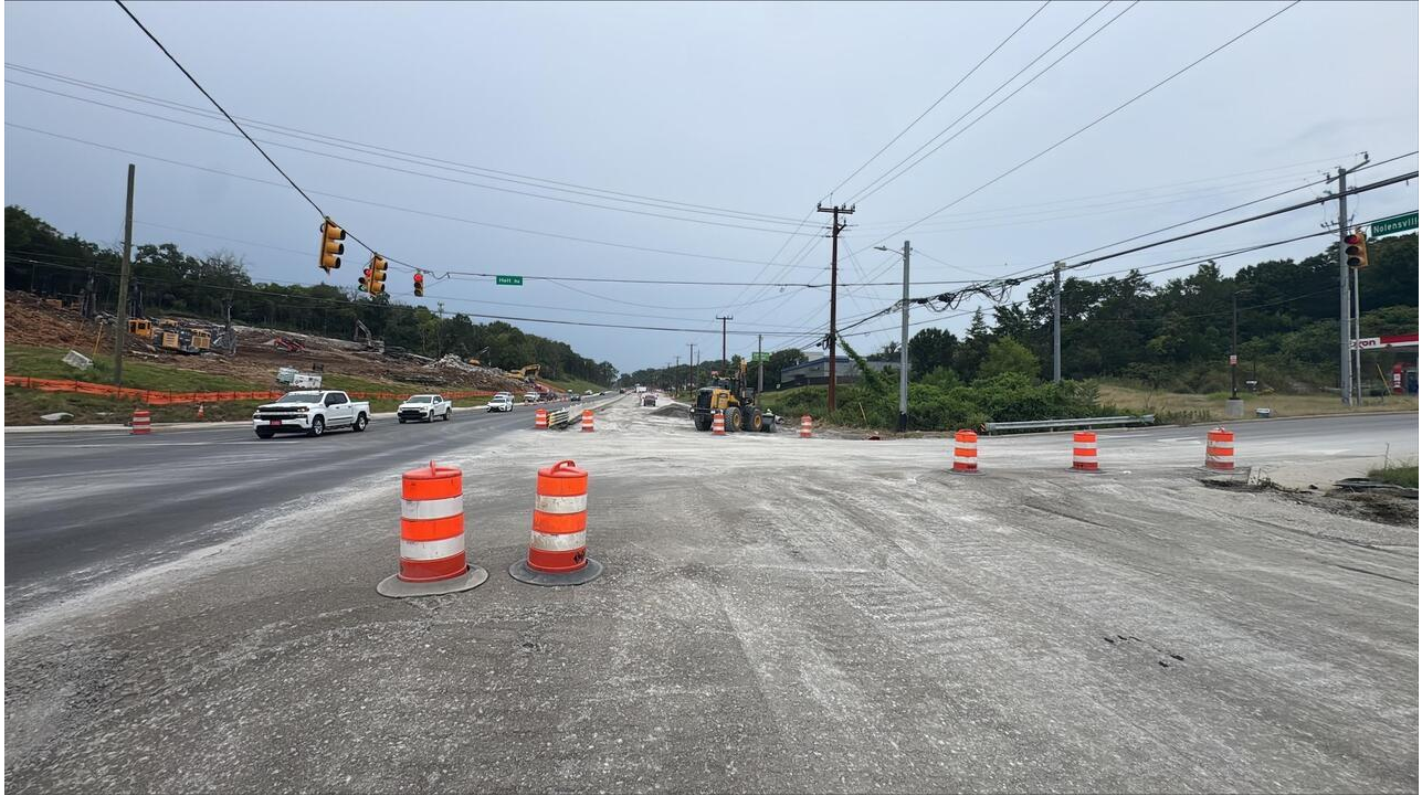
Base stone installation.
