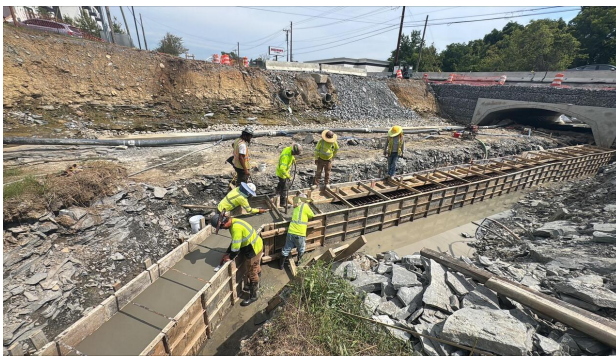
Mainline arch culvert placement.
