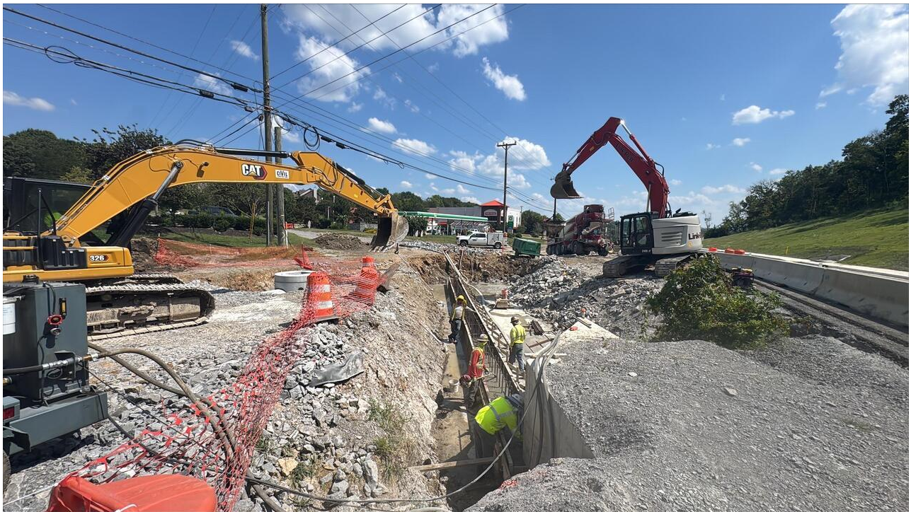
Box culvert placement.
