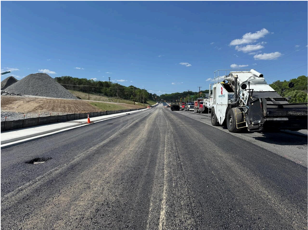
Main line paving.
