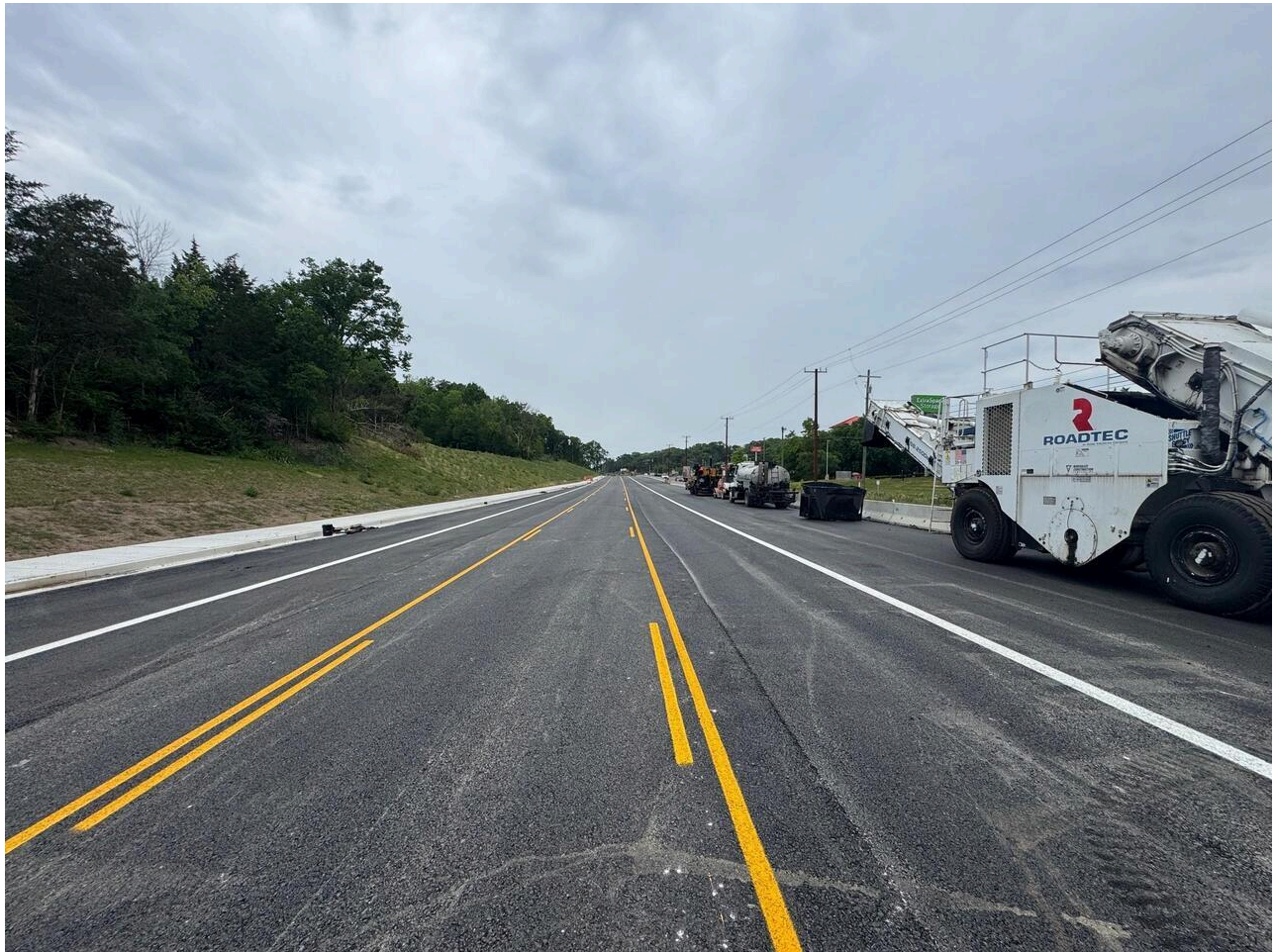
Striping for traffic shift.
