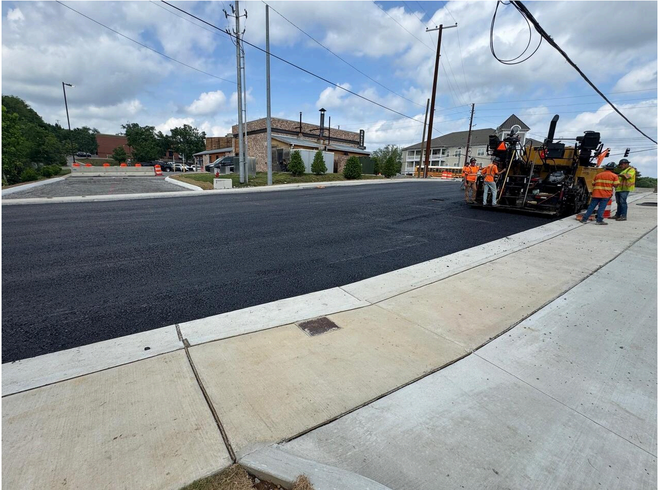
Bradford Hills Drive paving.
