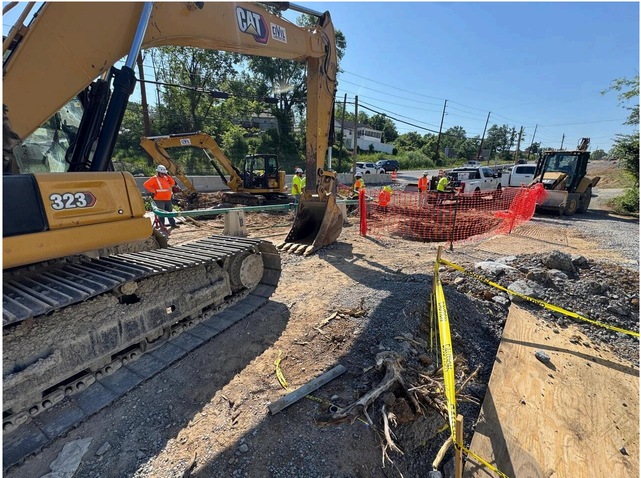
Gas line installation.
