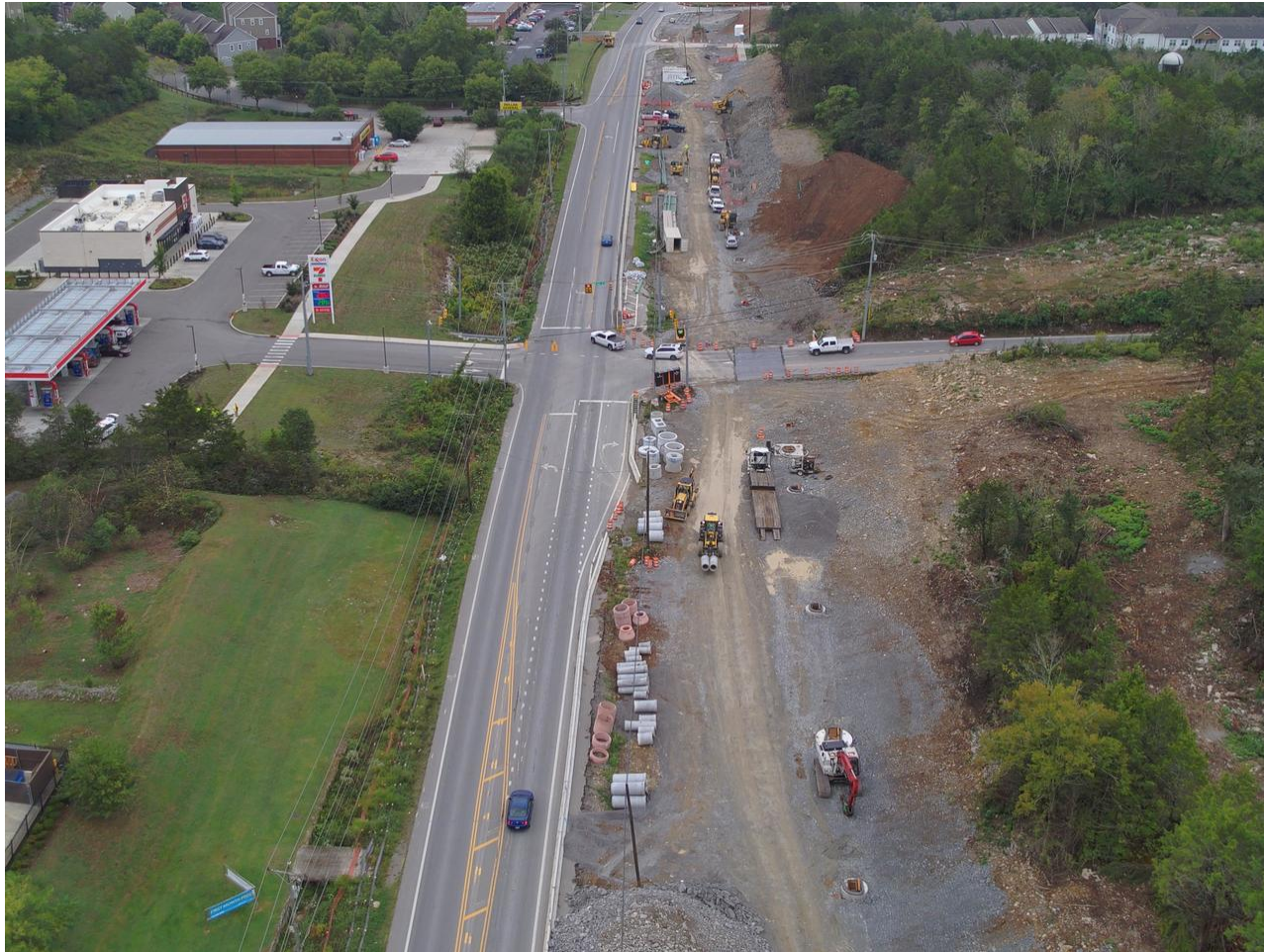
Utility work: Nolensville Pike near Holt Road looking south.
