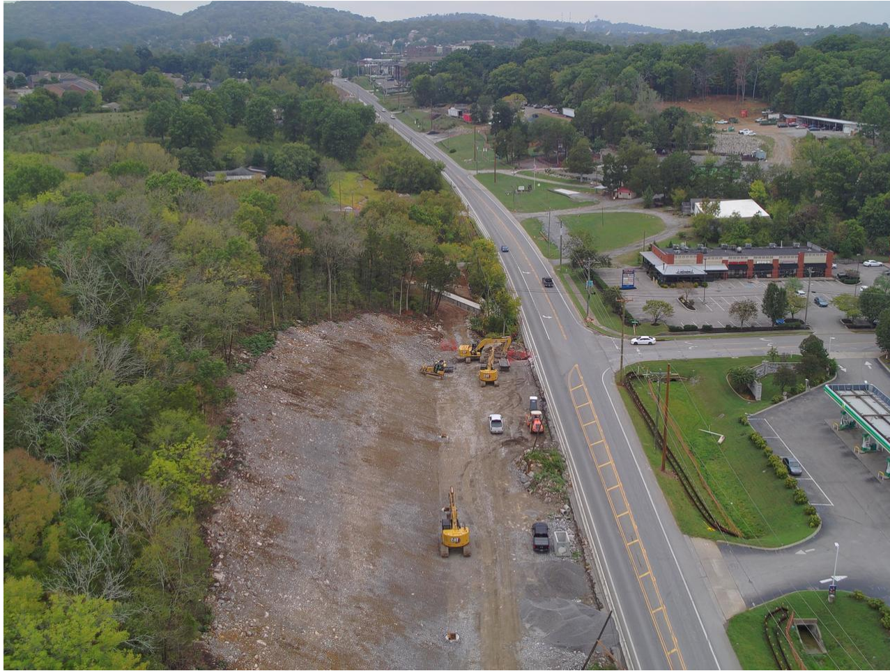
Gas line/utility prep: Nolensville Pike near Sugar Valley Drive looking north.
