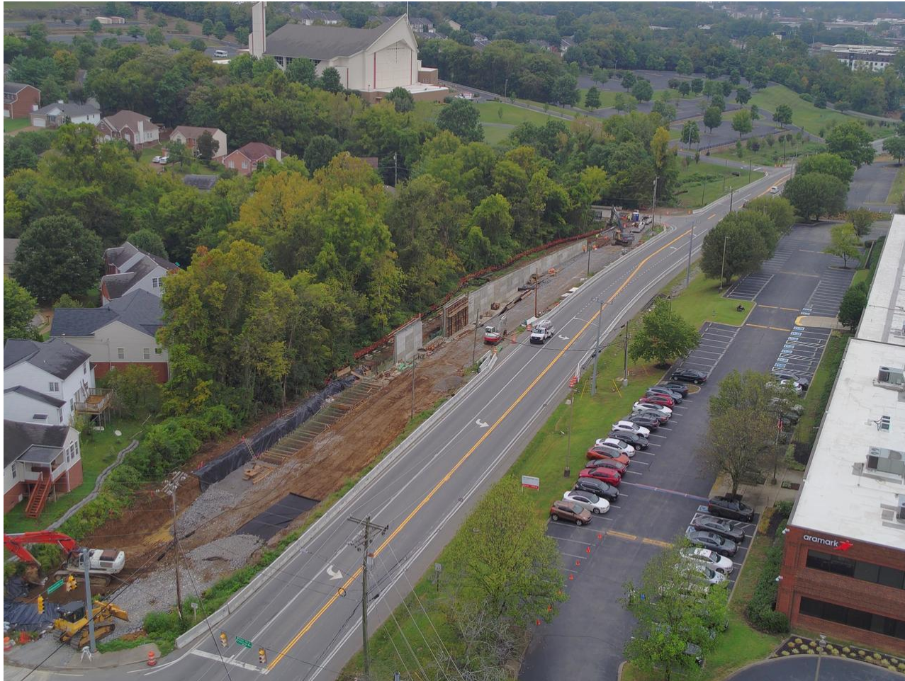
View of largest retaining wall in project: Nolensville Pike near Brentwood Highlands Drive looking north.
