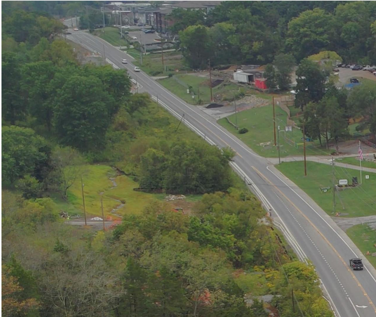
A closer look at the stream relocation.
