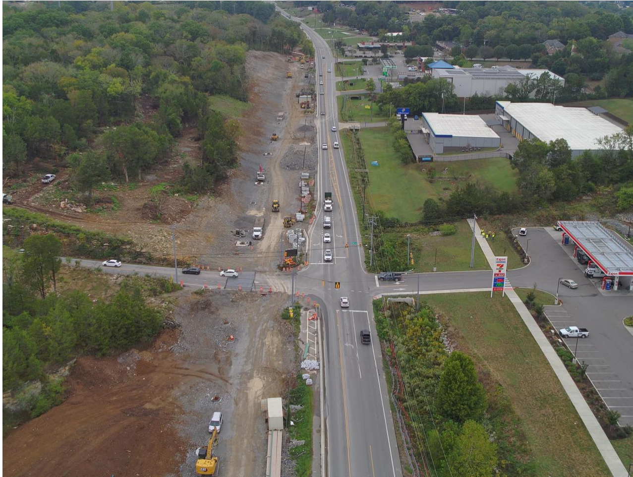
Water line preparation: Nolensville Pike near Holt Road looking north.
