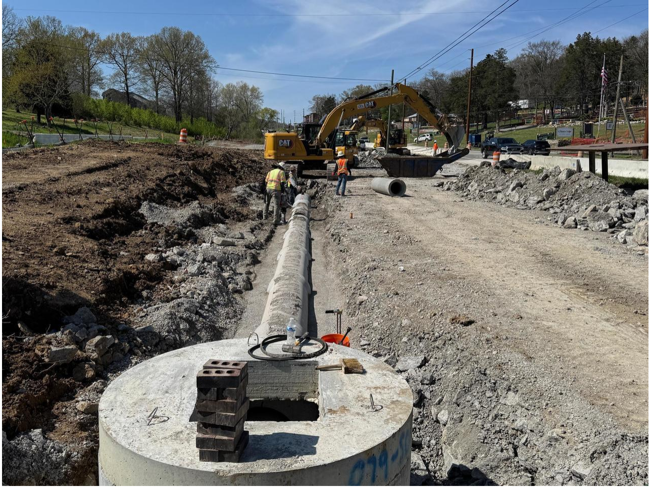
Storm drain installation.
