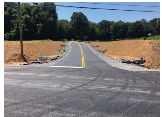
Completed work at Burton Road.
