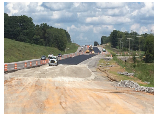
Paving at Bending Chestnut Road.
