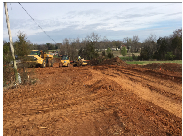
Grading work at the Academy Road intersection.
