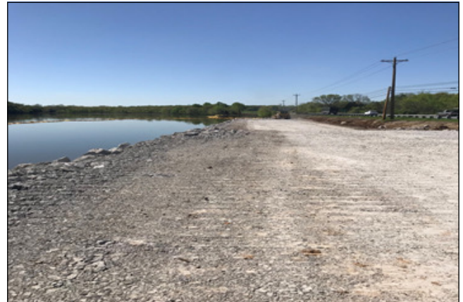
Graded solid rock at Dry Fork Creek
