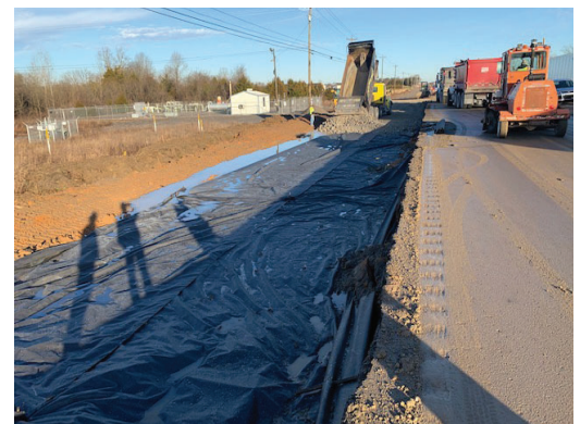
Subgrade work near Spence Creek Drive.
