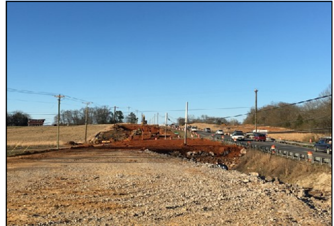
Grading at Tyree Access
