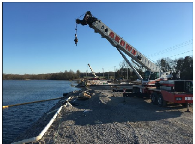
Parapet work at Dry Fork Creek Bridge
