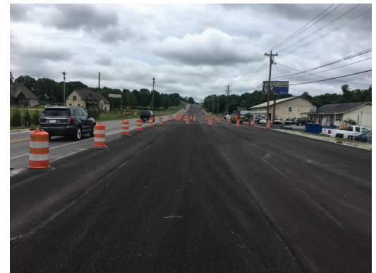
Paving at Wilson Road
