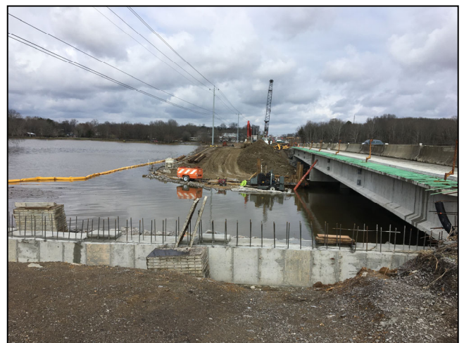
Bridge work at Dry Fork Creek
