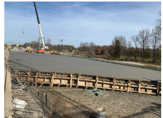
Bridge over Spencer Creek after concrete pour on November 24.
