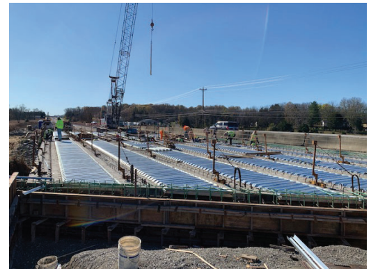
Bridge over Spencer Creek in early November.
