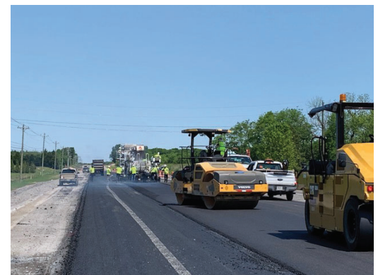
Asphalt base paving from Rock Castle Drive to Spence Creek Drive.
