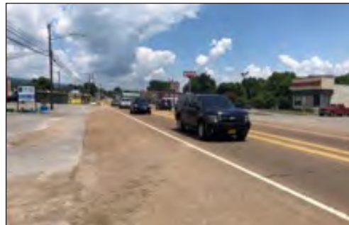
Figure 5: With no curb in the Project area, vehicles can enter the sidewalk at any place.
