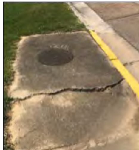
Figure 13: Sidewalks lack ADA-complaint crossings
