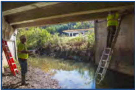
Bridge Repair Field Inspection
