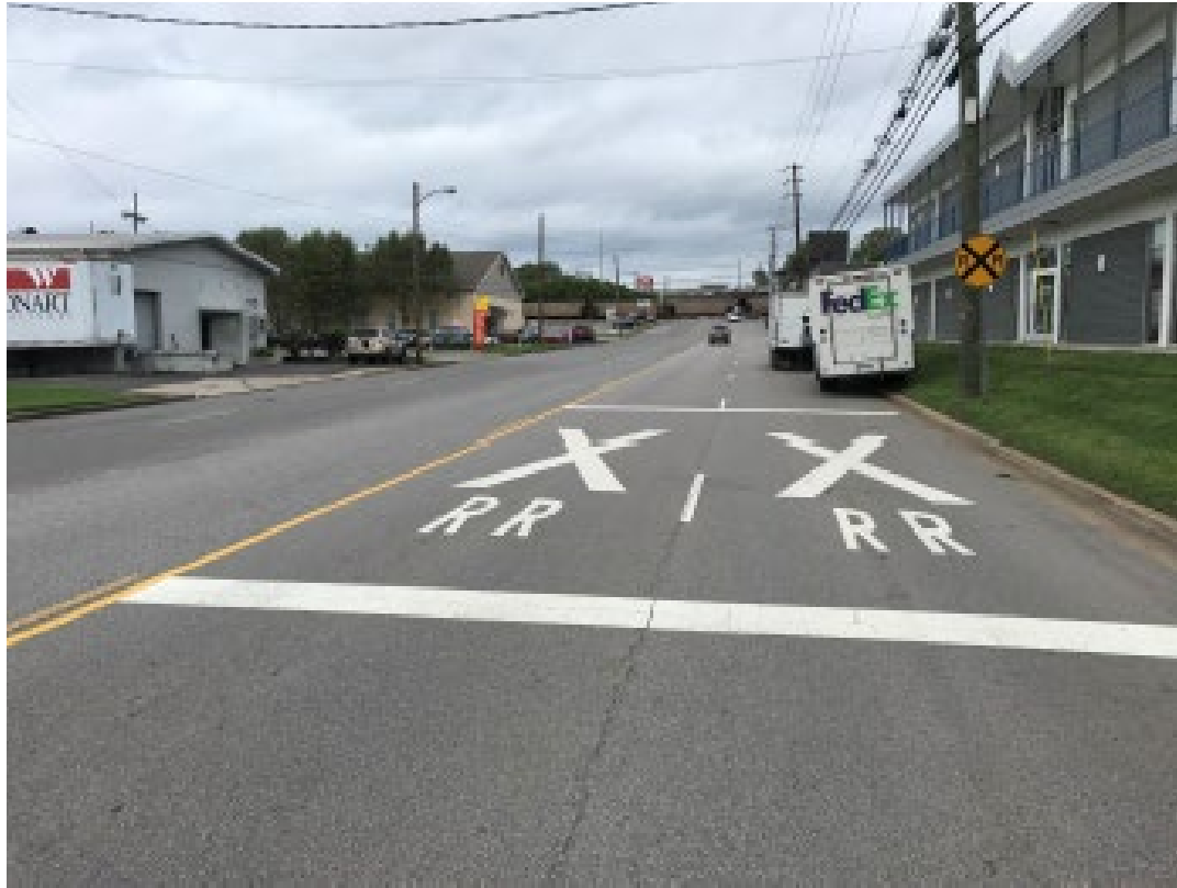
#8 – Advance warning signs and pavement markings
