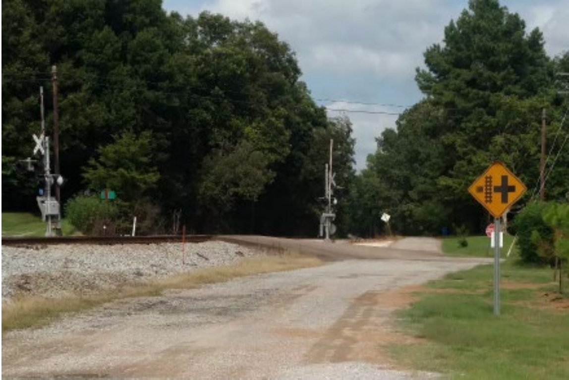
#10 - Warning signs on parallel roads
