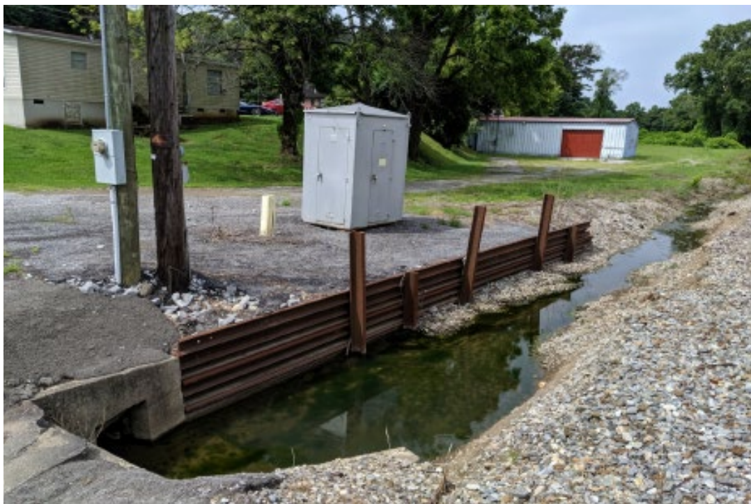
#9 - Adjacent drainage features
