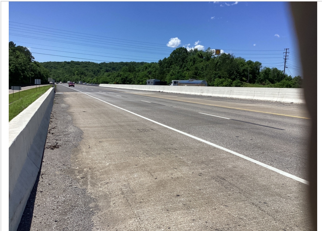
R view across deck B to A
