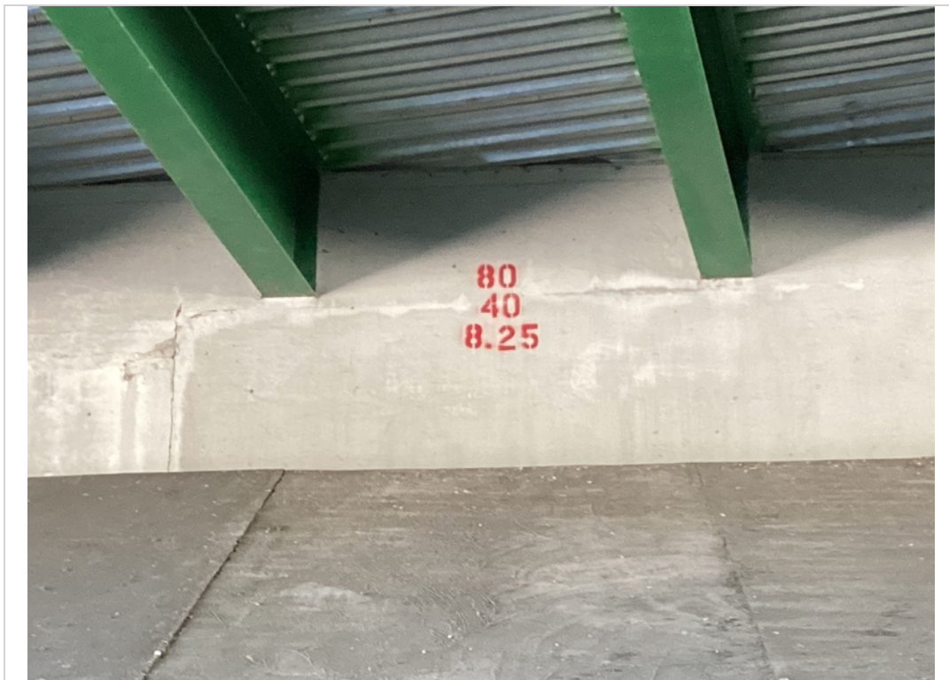
Bridge number abutment 1 mid
