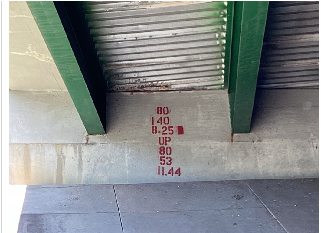
Bridge and up number abutment 1 right
