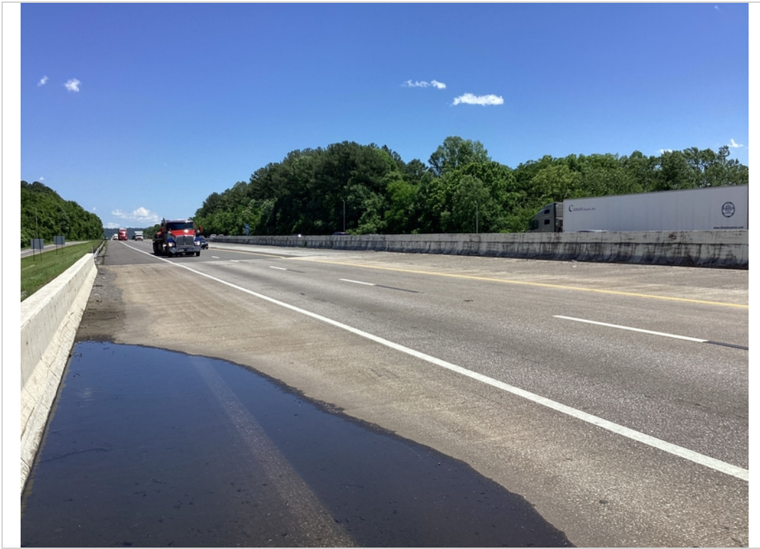
L view across deck
