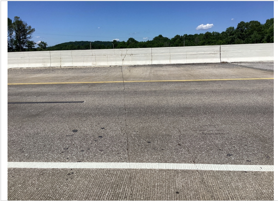
R B approach joint span 3
