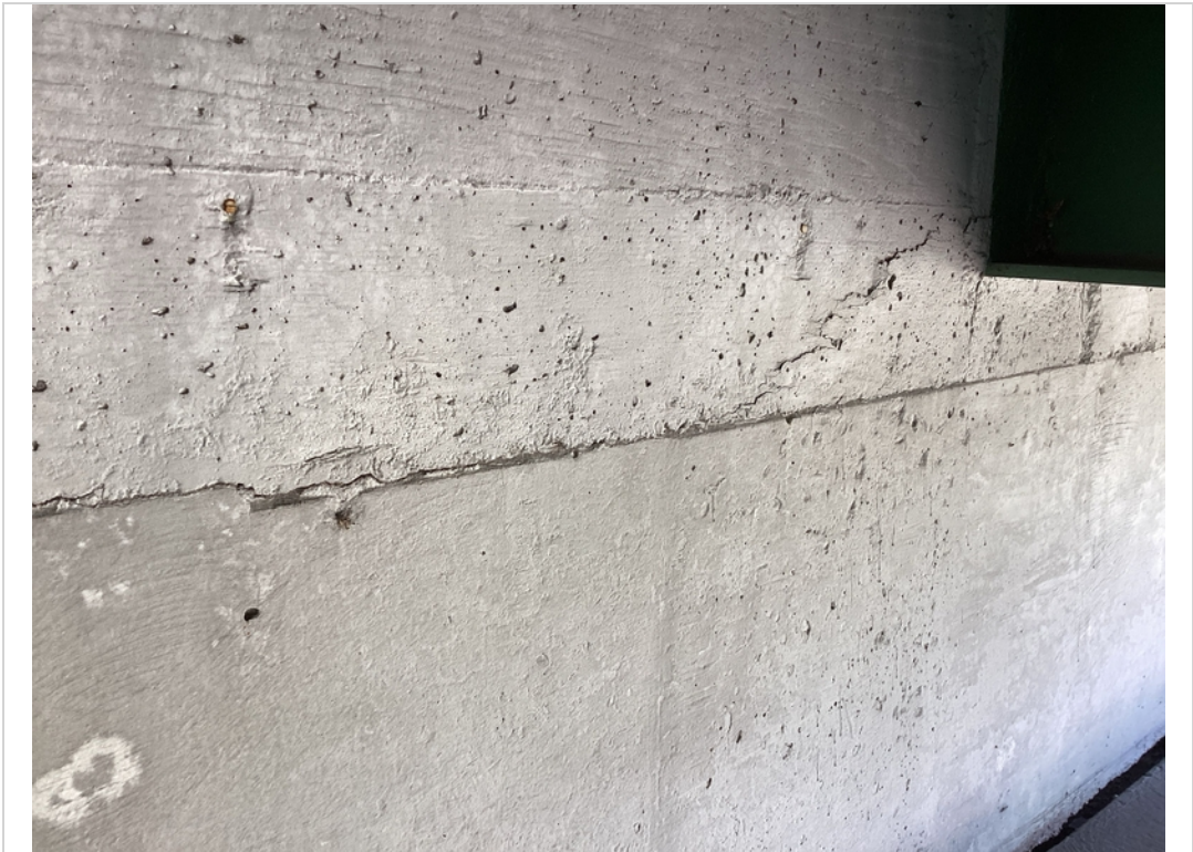
Abutment 2 backwall bay 17 Hc
