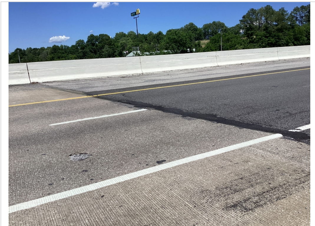
R B approach joint span 3
