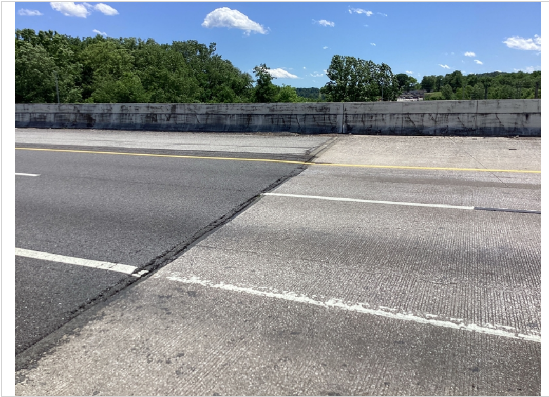
L B approach joint span 3
