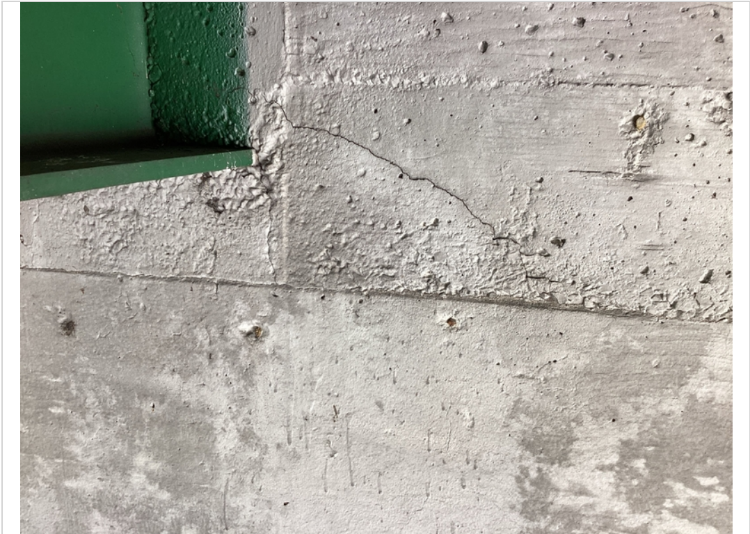
Abutment 2 backwall bay 17 Hc
