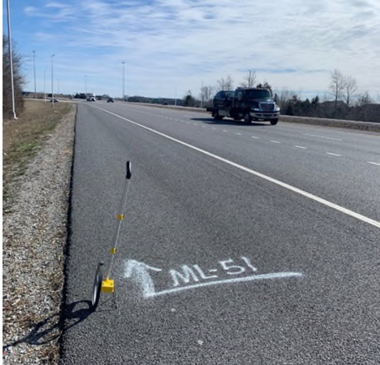
Figure 1: Segment Identification Marking
