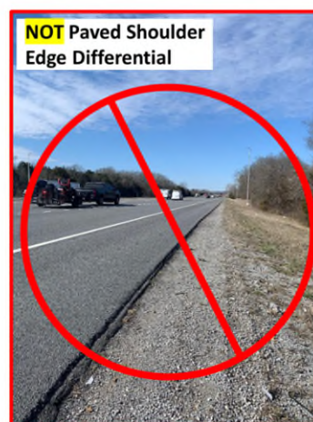
Any change in elevation between the pavement and unpaved shoulder should be evaluated as Unpaved Shoulder Drop-Off.
