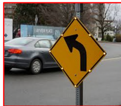
This image depicts functional warning lights
