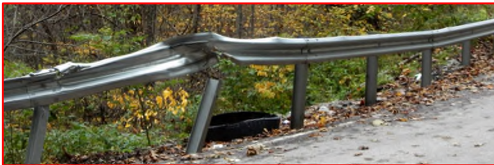
Deficient guardrail
