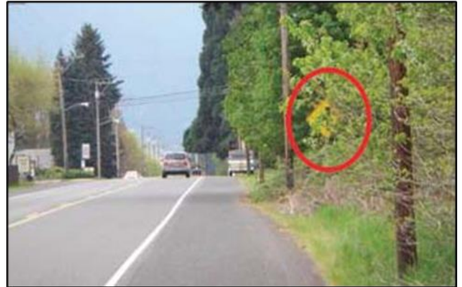
Example: Sign obstruction.
