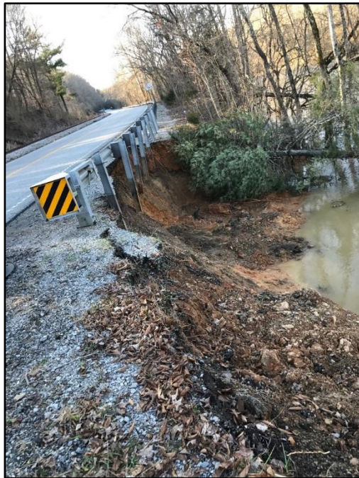
Examples: Slope with > 6-inch deviation in depth.
