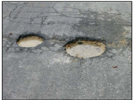
Pothole examples - greater than 6 inches in diameter and 1.25 inches deep, failing the criteria.
