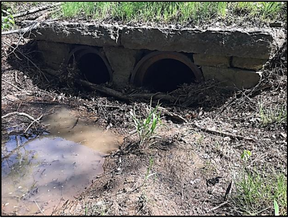
Example: Less than 50% of structure is blocked.
