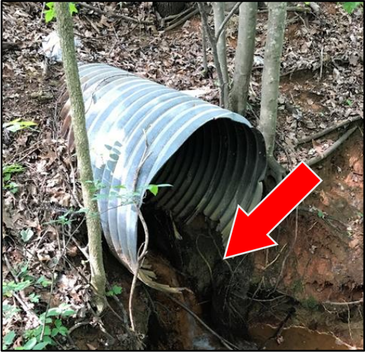
Example: Eroded area around inlet is greater than 1.5 times the diameter.
