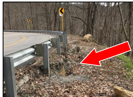
Examples: Slope with > 6-inch deviation in depth.
