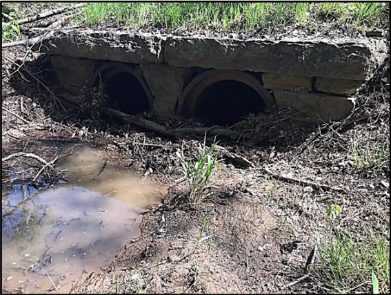
Example: Less than 50% of structure is blocked.
