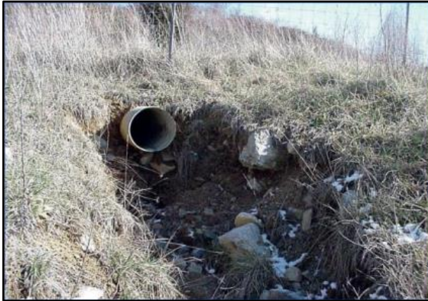
Example: Eroded area around inlet is greater than 1.5 times the diameter.
