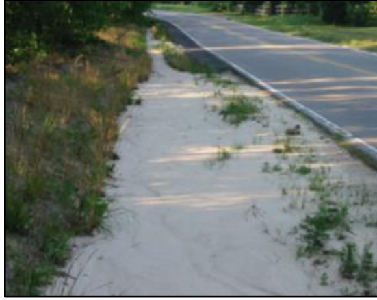
Examples: Left - Ditch with less than 50% blockage. Right – Ditch with greater than 50% blockage.
