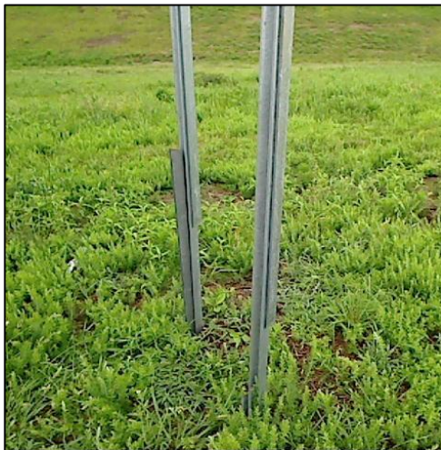
Example: This u-channel post is lapped onto the previous sign mount which creates a greater than 3 lbs/ft weight without a breakaway assemble and does not meet the desired condition.
