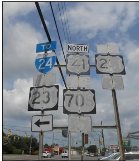
Example: Faded sign with sign face missing damage.
