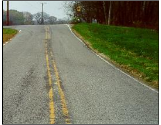
Example: Striping faded.
