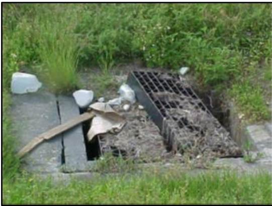
Example: Grate is out of the cradle.
