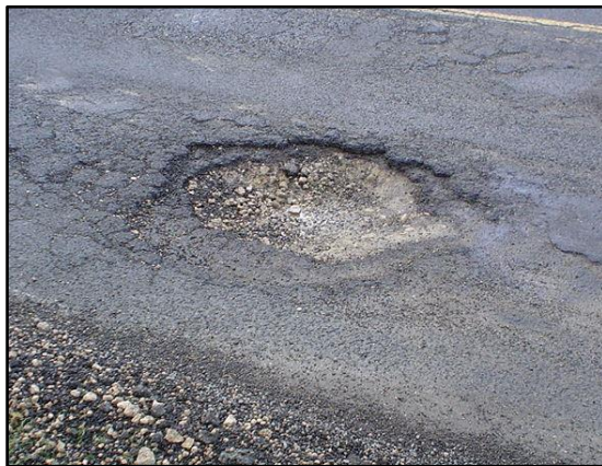
Pothole examples - greater than 6 inches in diameter and 1.25 inches deep, failing the criteria.
