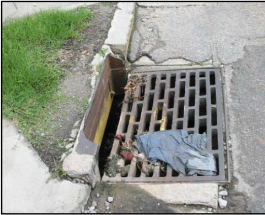
Example: An inlet that has approximately less than 50% blocked would meet the threshold condition.
