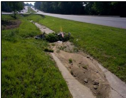
Example: Paved ditch with >50% of depth blocked by debris for 50 continuous feet.
