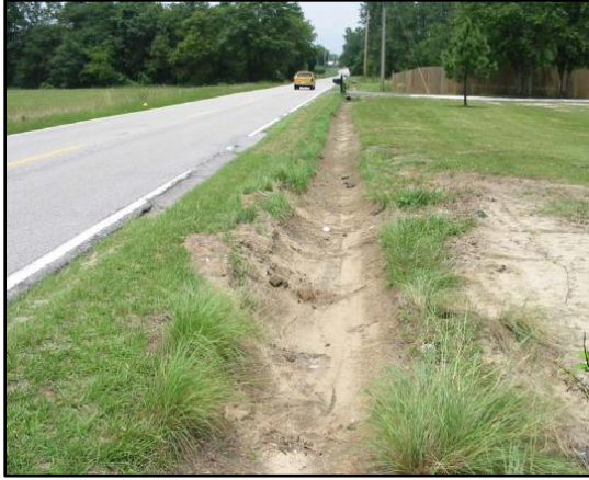
Examples: Left - Ditch with less than 50% blockage. Right – Ditch with greater than 50% blockage.
