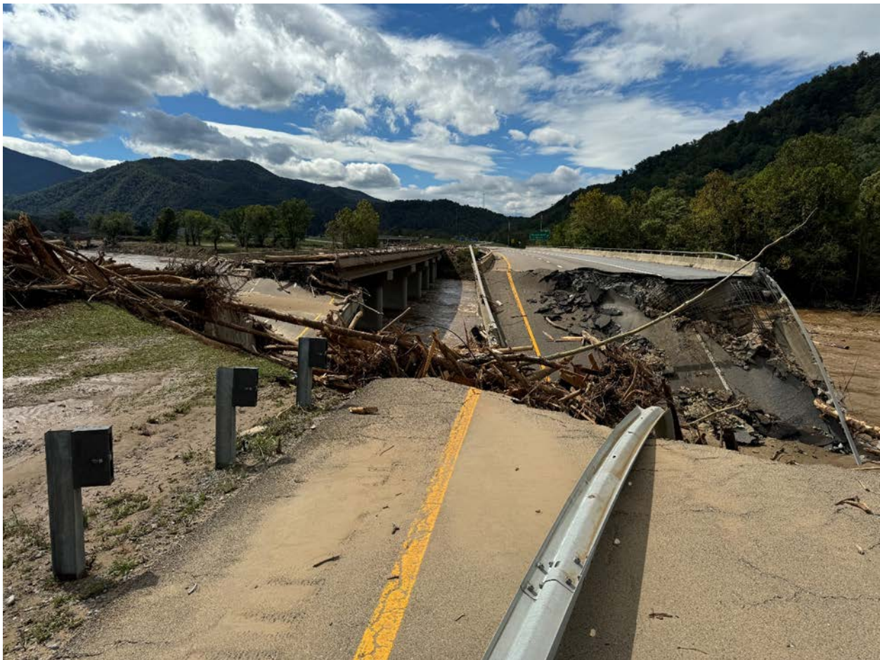
Figure 5-6: Damage on I-26 in Unicoi County that occurred because of Hurricane Helene
