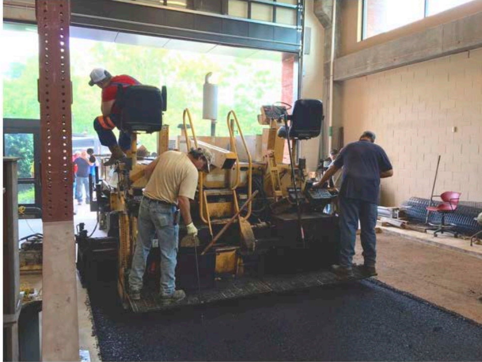
Figure 5. Paving of the Asphalt Mixture in the Test Pit
