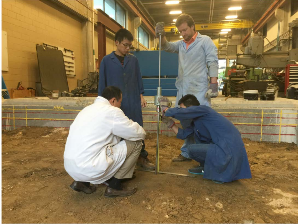
Figure 3. Testing the Density of the Subgrade Using Dynamic Cone Tester
