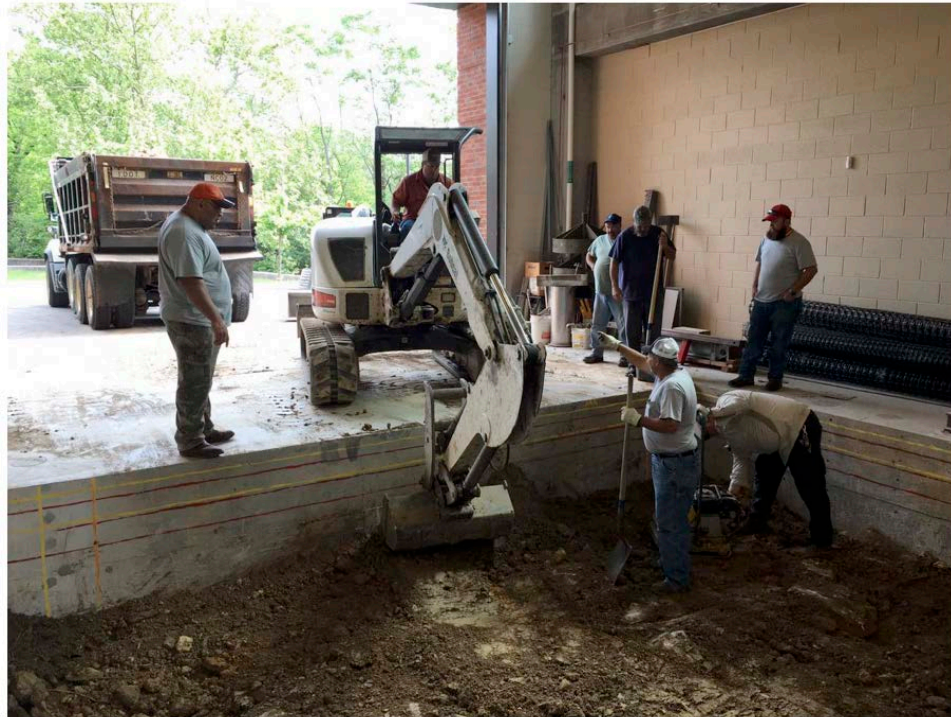
Figure 4. Construction of the Subgrade in the Test Pit
