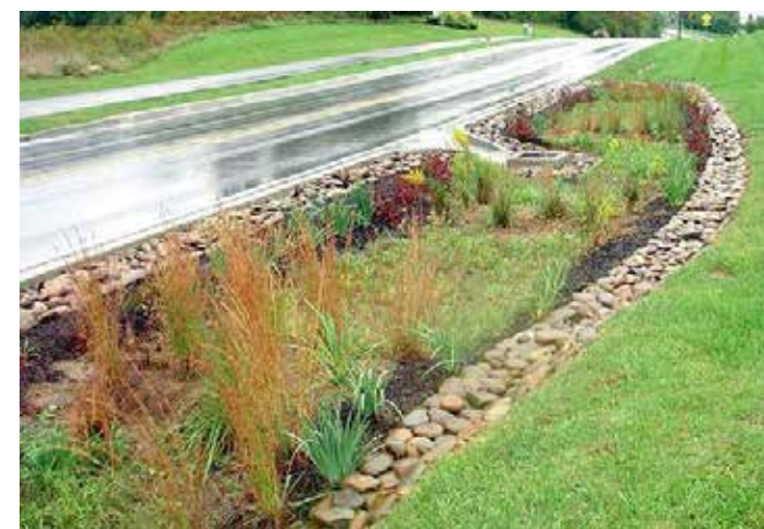
Typical Road Section with pedestrian pathway, landscape enhancement, and integrated storm water management.
