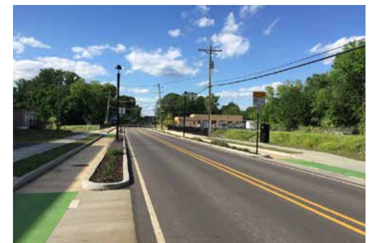
Typical Road Section with protected bike and pedestrian pathways and, intentional signage and lighting design.
