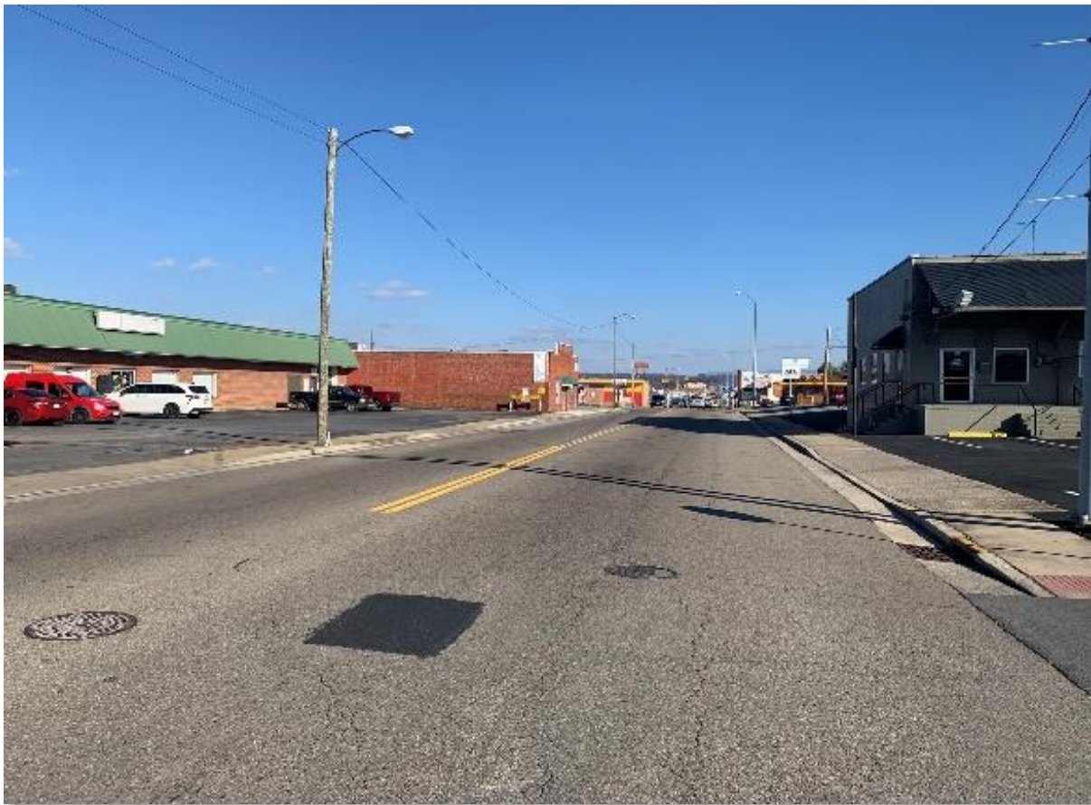
Segment 2 is characterized as a 2-lane roadway with frequent driveways and sidewalks.
