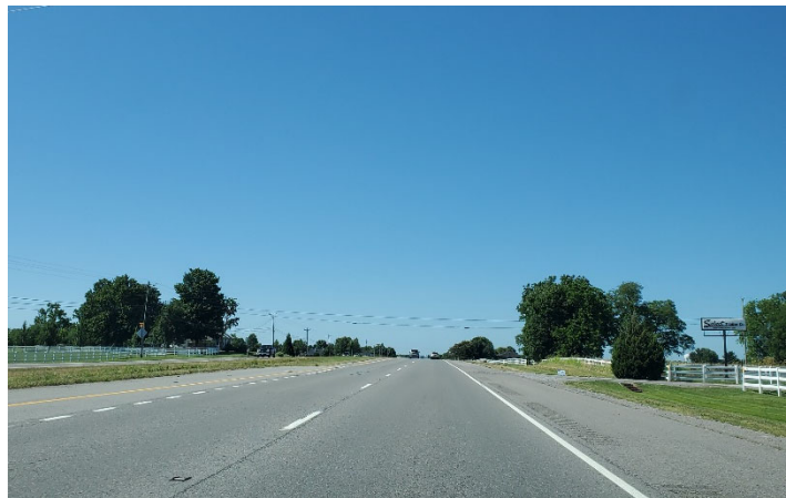
US 231 South of Eady Road/Webb Highway /SR 82 Intersection (Southbound)
