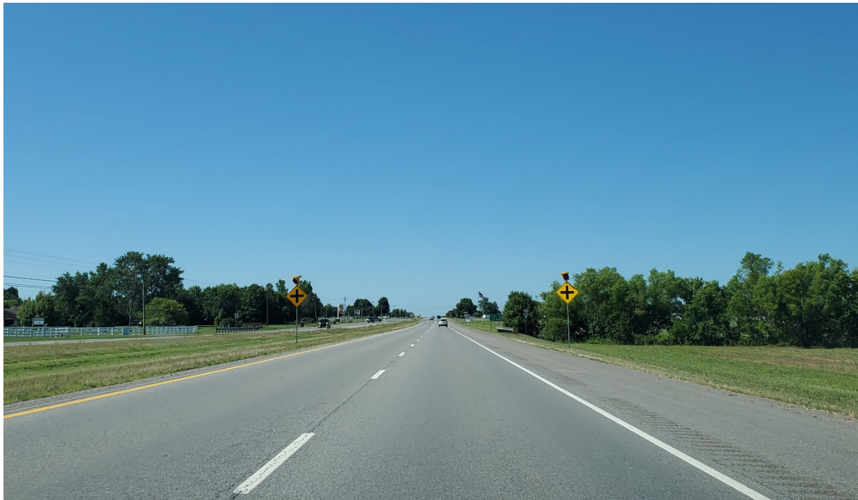
US 231 Approaching Eady Road/Webb Highway/SR 82 Intersection (Southbound)
